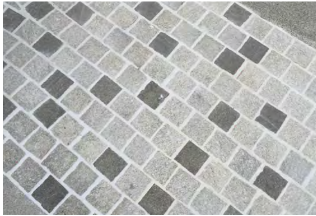
Stone Setts Pavement
