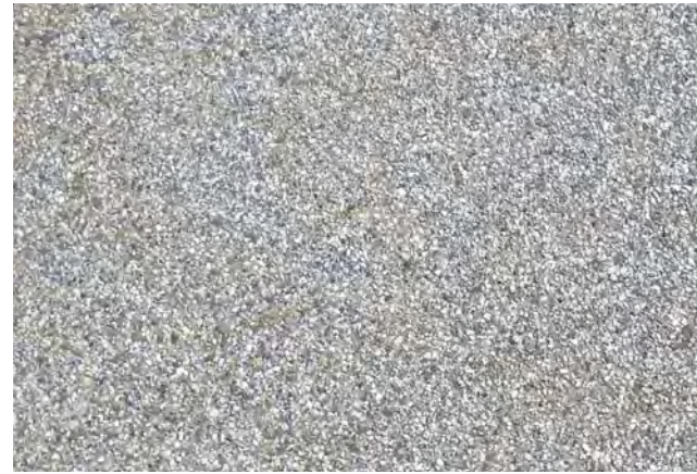
Exposed Aggregate Concrete Pavement
