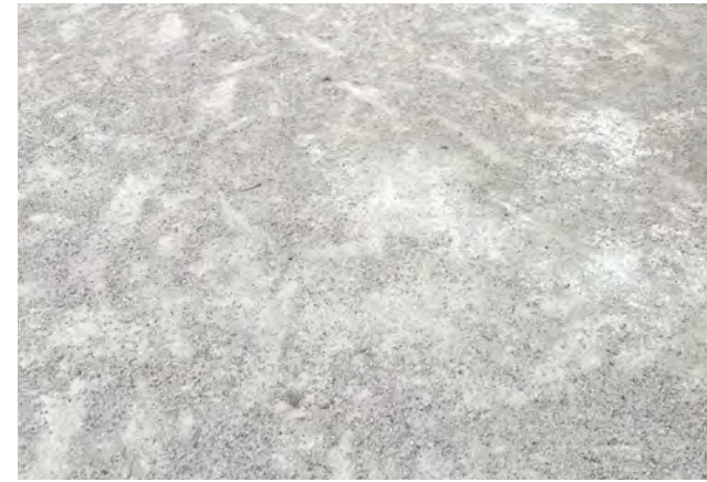
Decomposed Granite Pavement
