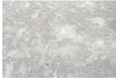
Decomposed Granite Pavement
