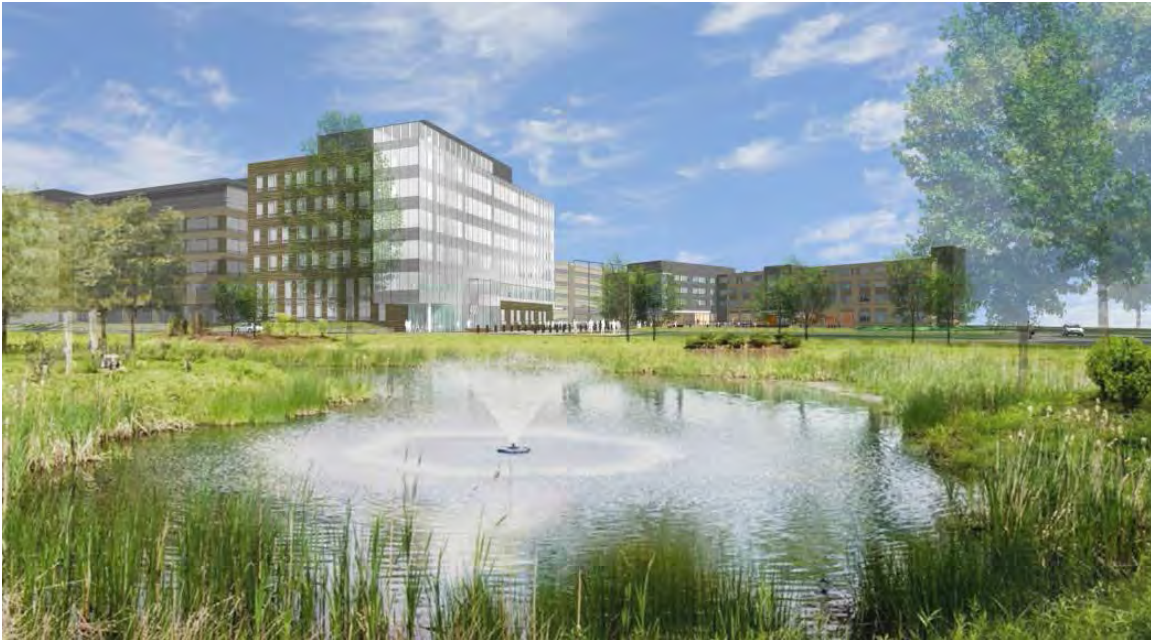
Image of eastern facade of stand-alone Building 400
