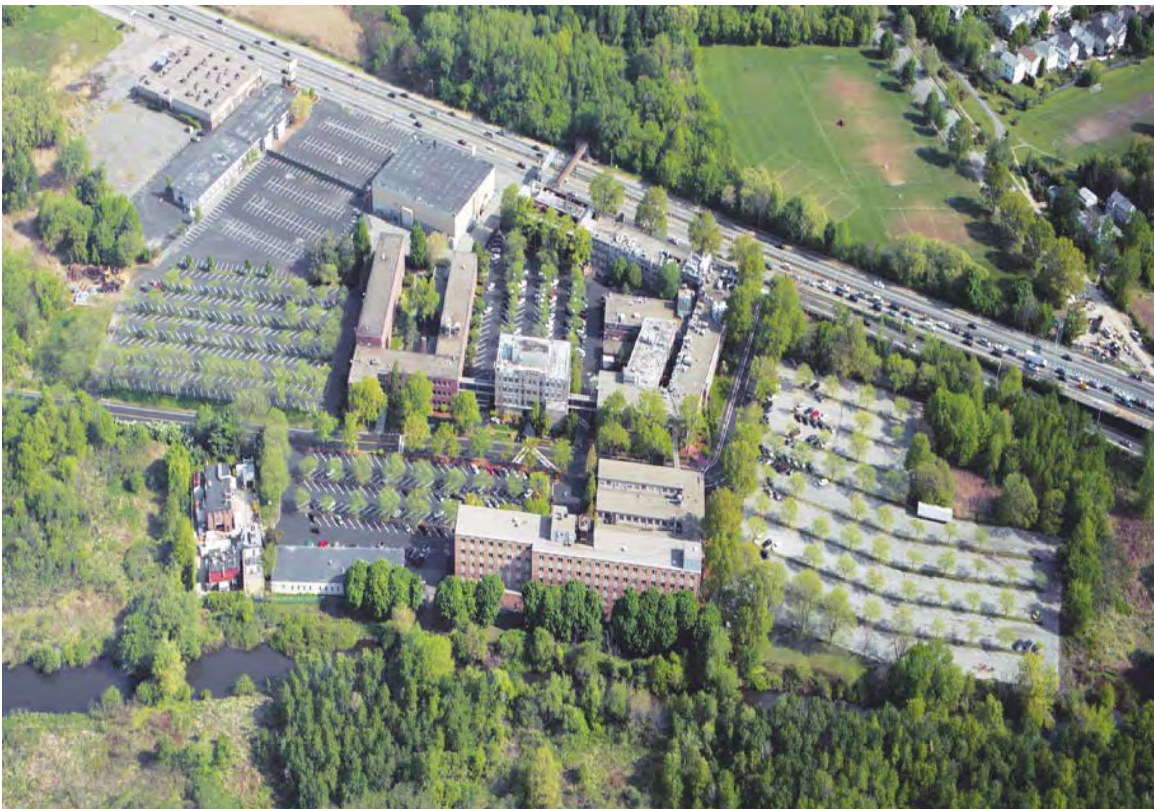
Aerial view of former ADL Campus, circa 2000
