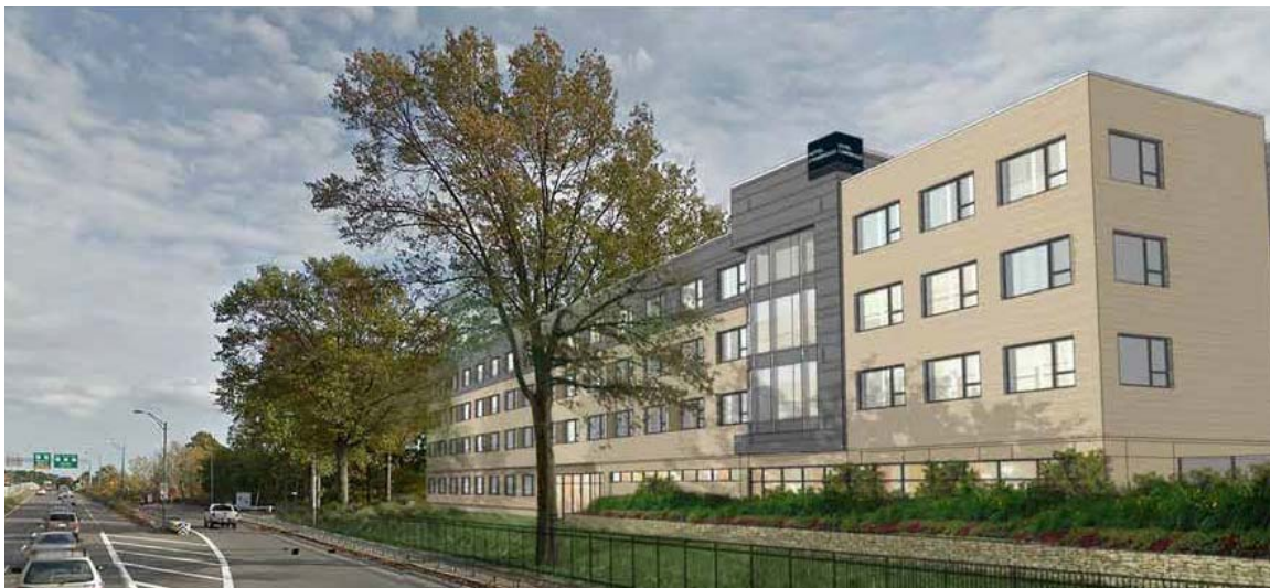
View of north side of hotel from Route 2 Alewife exit ramp.
