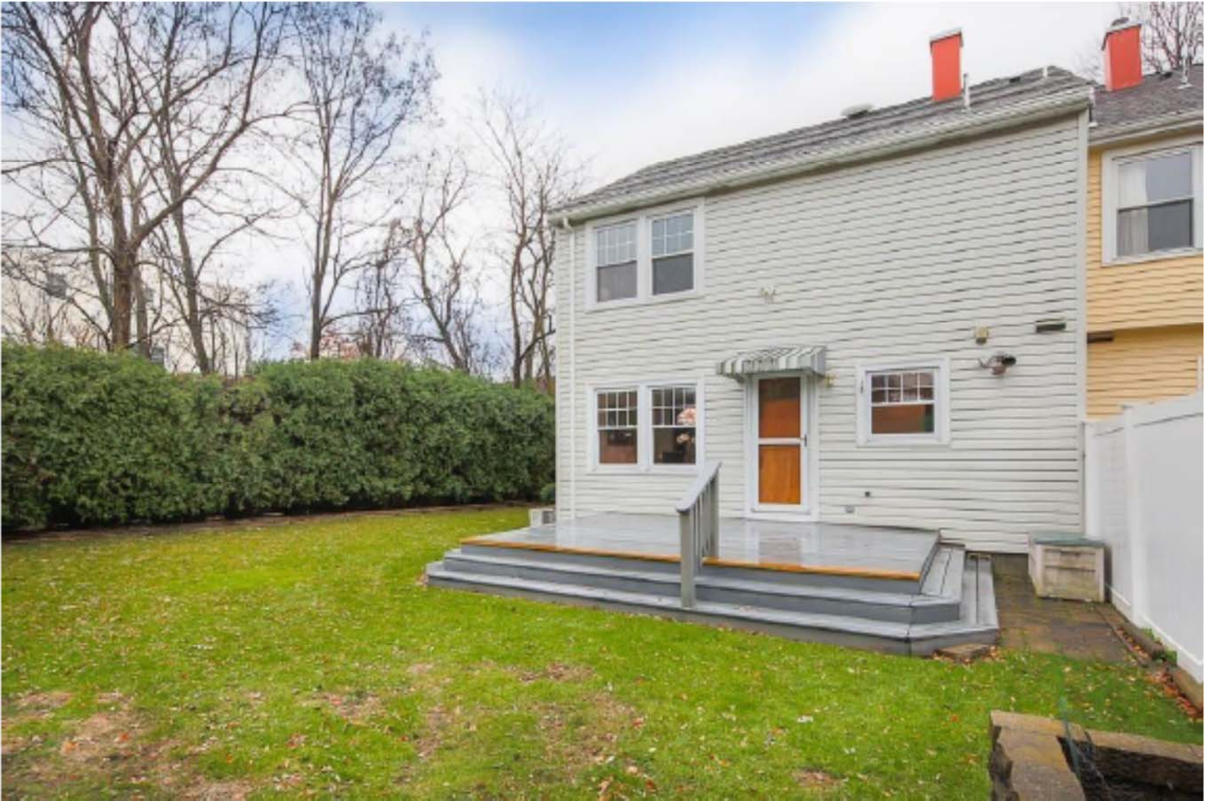
16 James Way Cambridge MA Existing Condition Photograph-Back View
