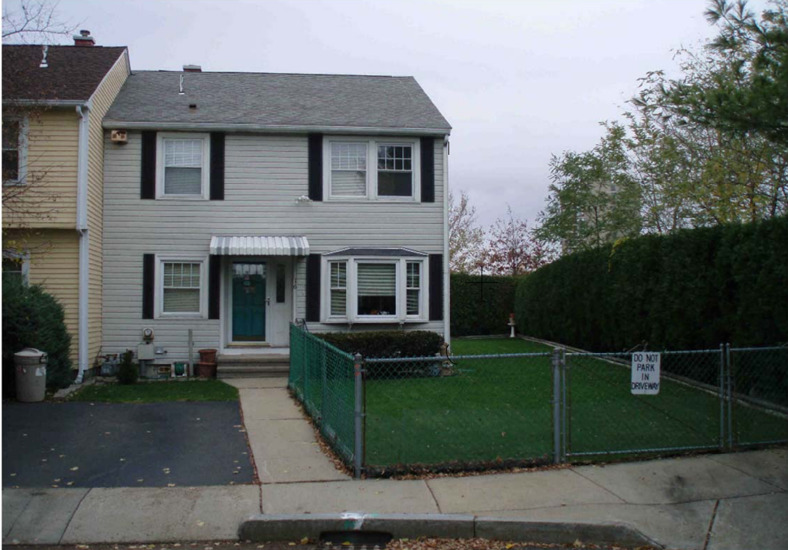
16 James Way Cambridge MA Existing Condition Photograph-Front View
