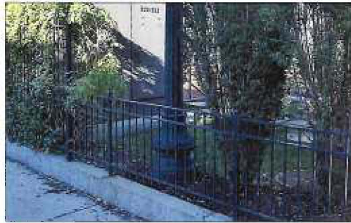
Steel Picket Fence at Veritas Hotel
