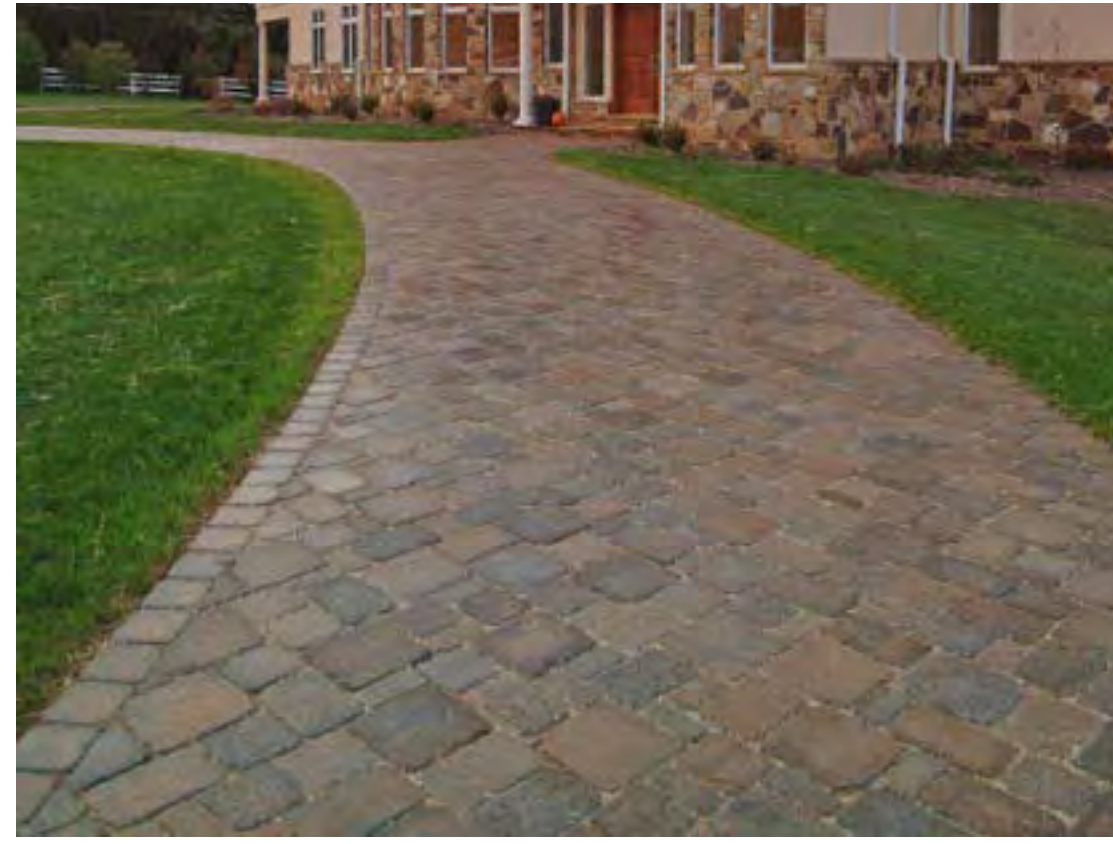
CONCRETE UNIT PAVING
