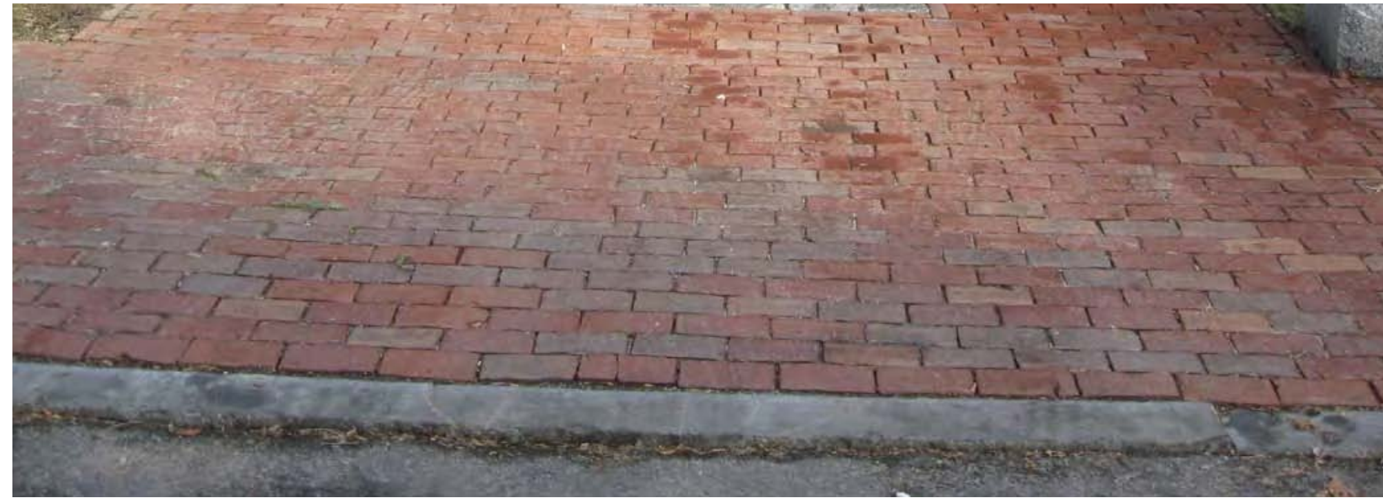
BRICK PAVING - RUNNING BOND PATTERN
