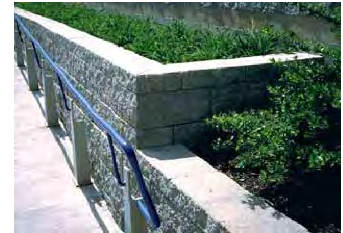
CONCRETE UNIT BLOCK RETAINING WALL
