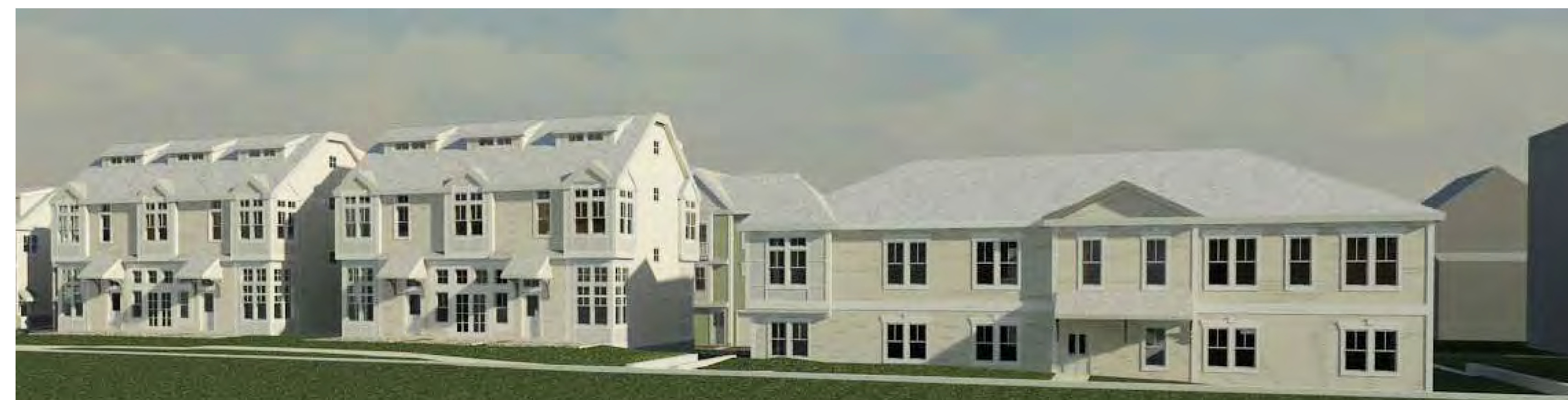
VIEW OF UNITS 13 TO FLATS FROM BIKE PATH
