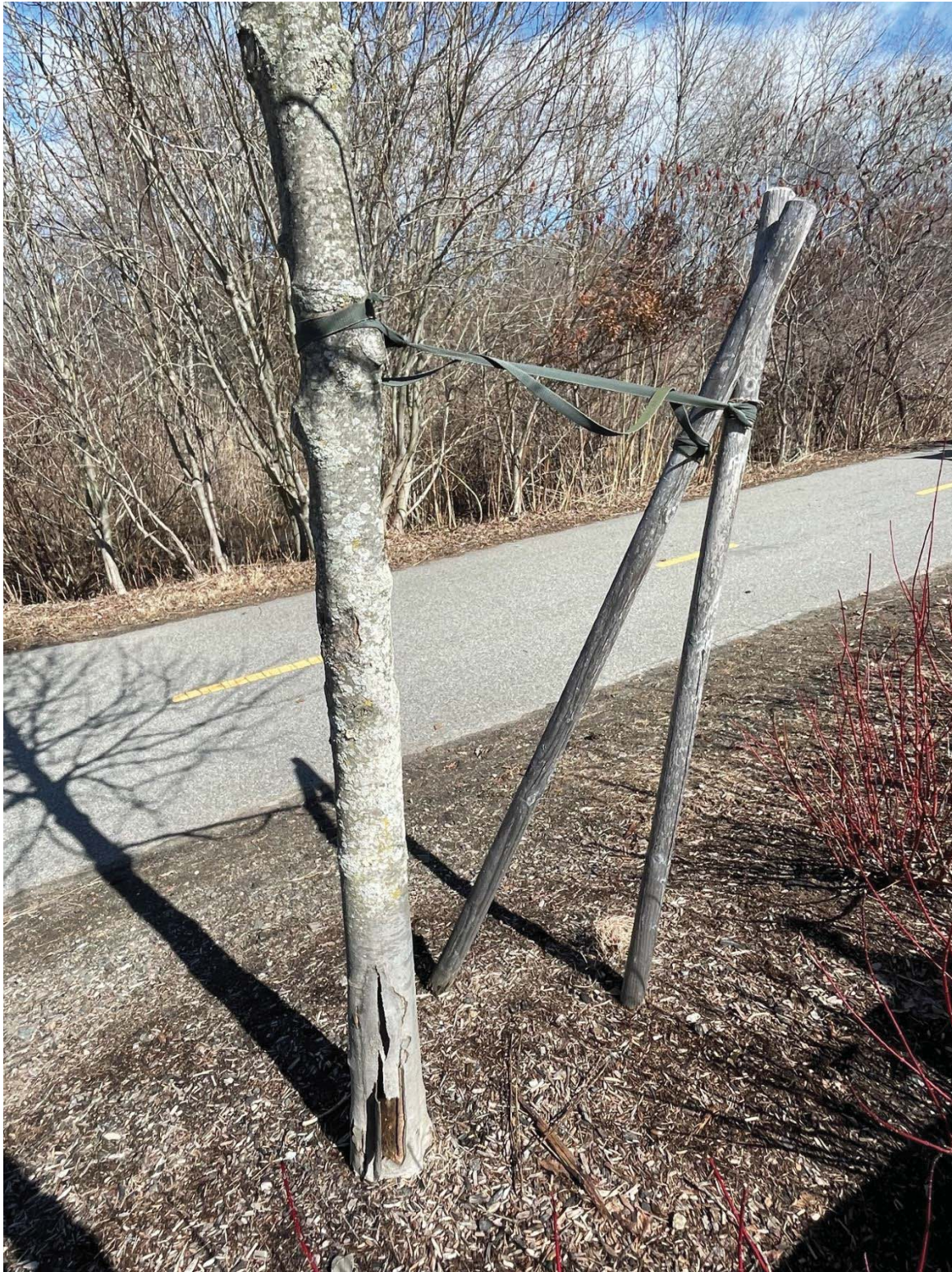
Tree #28 exhibiting a lower stem wound and a buried root collar. Planting material was also noted; guys should be removed from the young tree before the stem grows too large and the staking material begins to girdle the tree. In this example, one side of the guy system is already broken and just leaning against the other so the system as a whole is not achieving the intended purpose.
