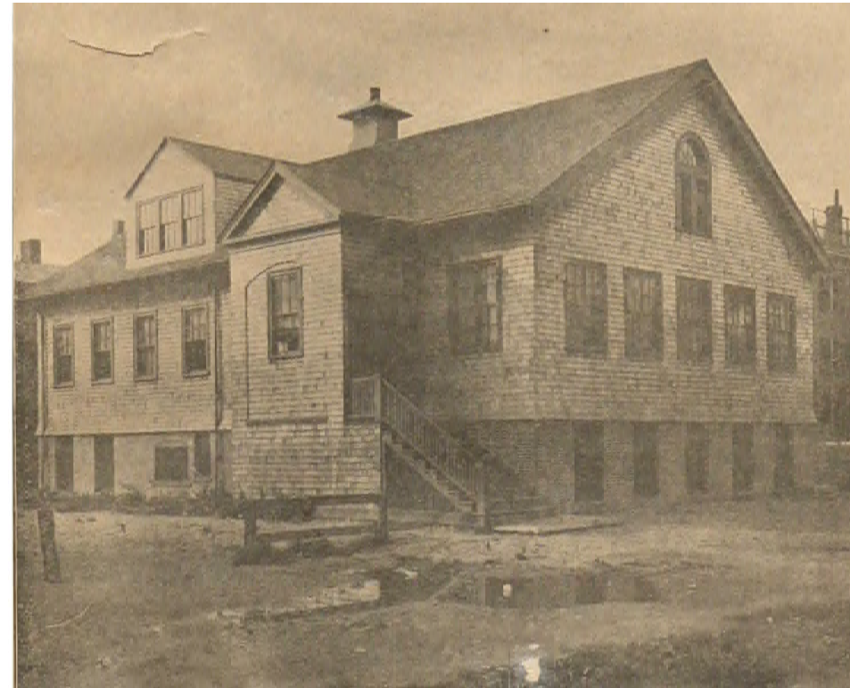
RIVERSIDE ALLIANCE BUILDING, BALLORD PLACE PHOTO CIRCA 1910
