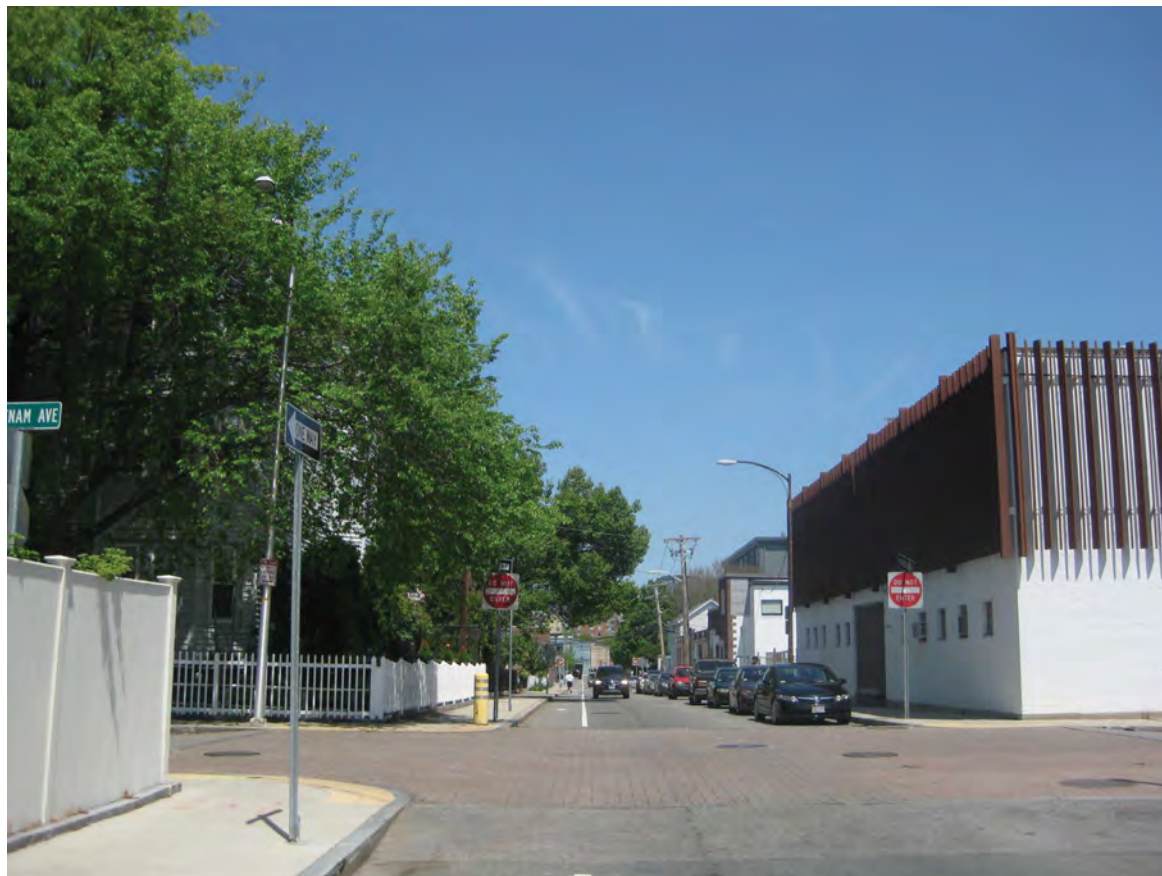
EXISTING - SIDNEY STREET LOOKING NORTH
