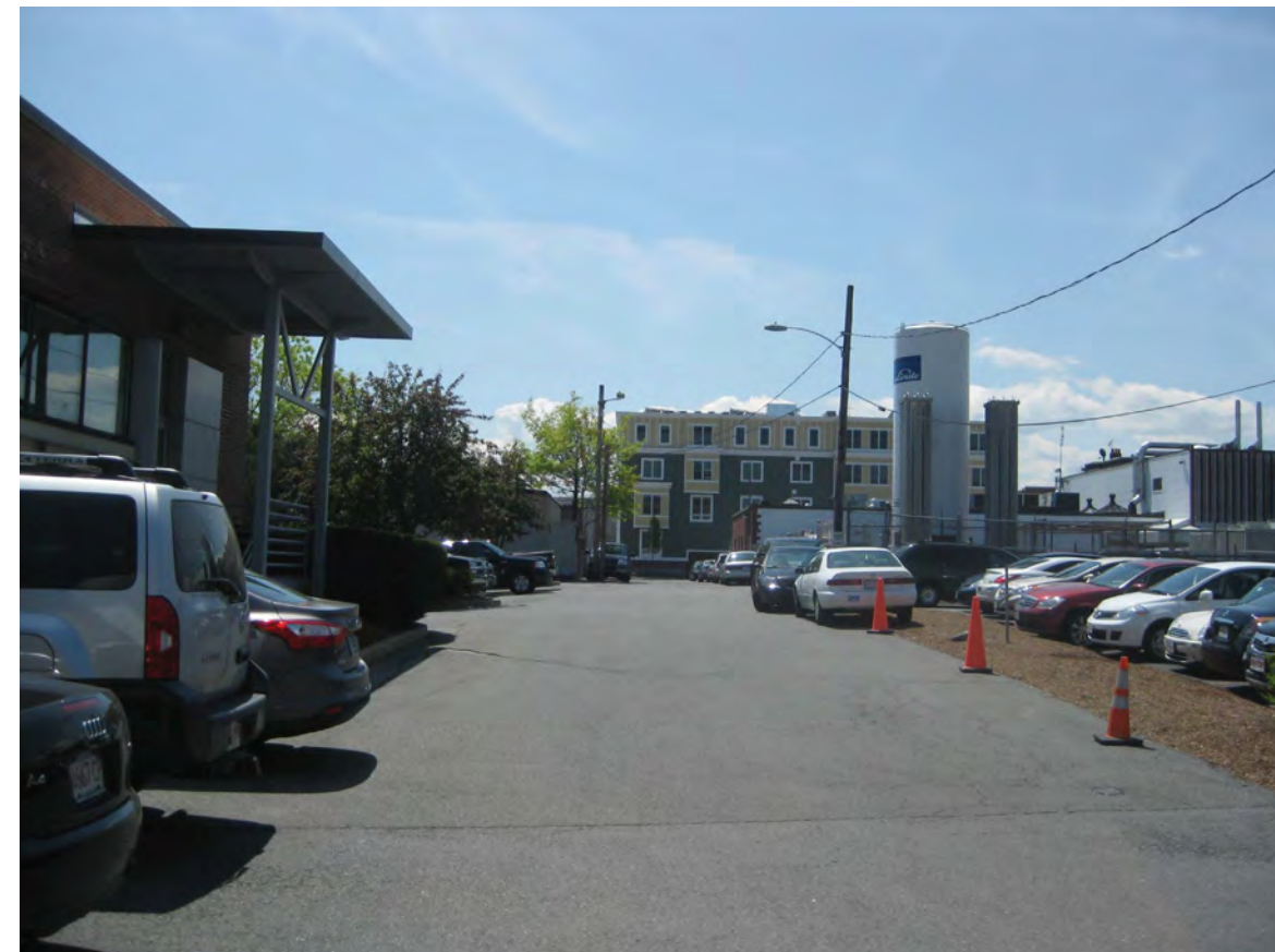
EXISTING - GROVE STREET LOOKING SOUTH
