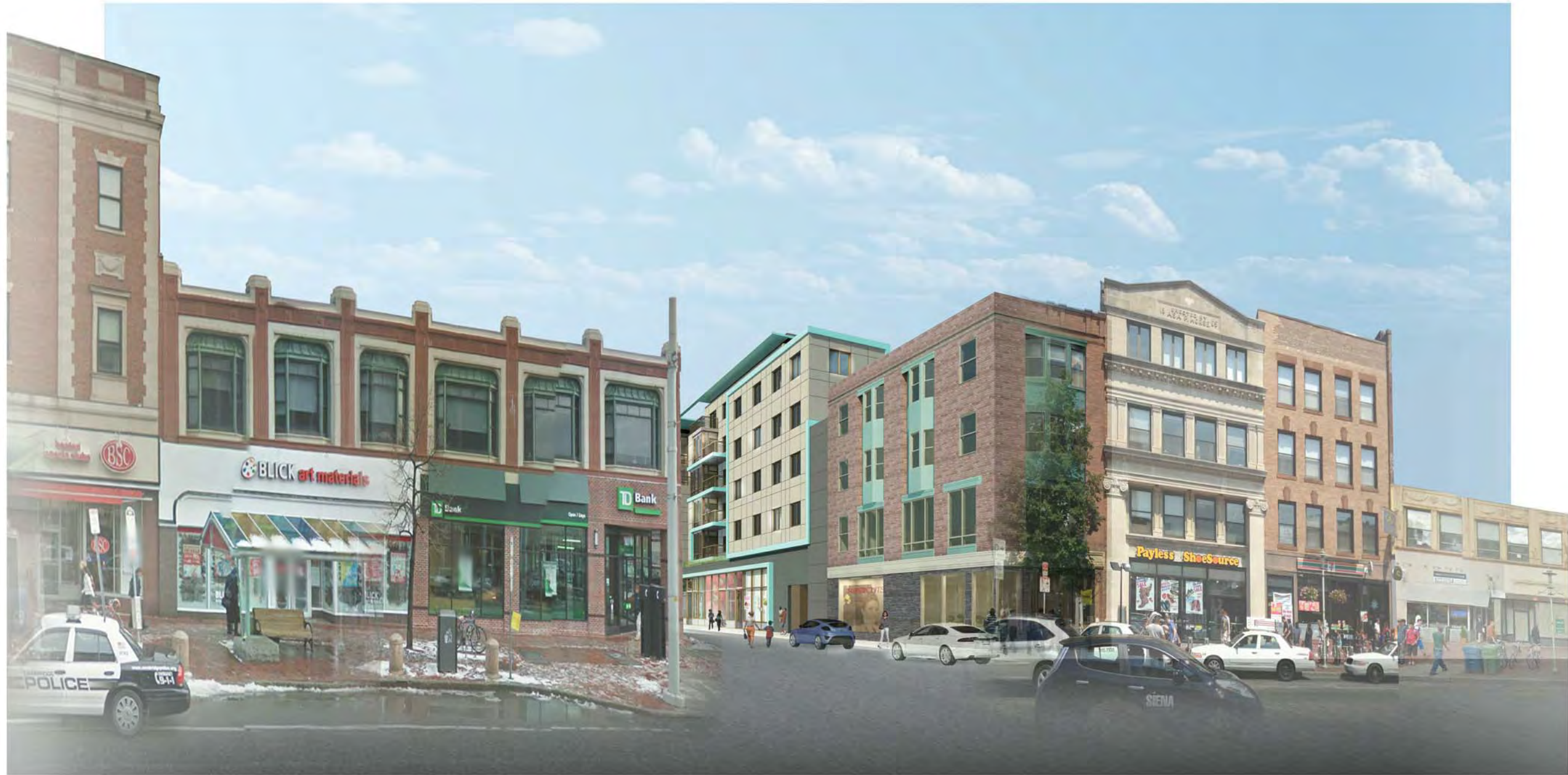
VIEW FROM MASSACHUSETTS AVE.
