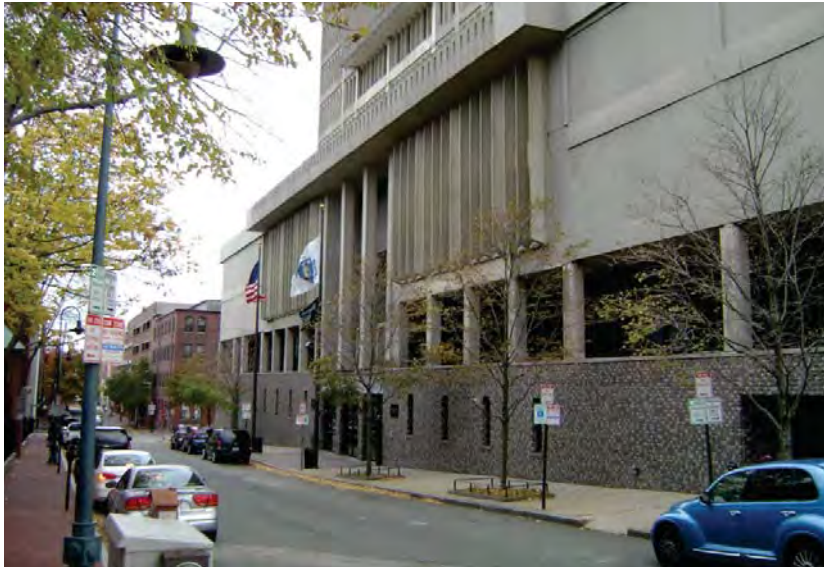
10. VIEW FROM THIRD ST TOWARD THORNDIKE ENTRANCE
