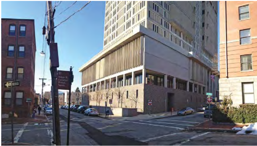
3. SECOND STREET & THORNDIKE STREET
