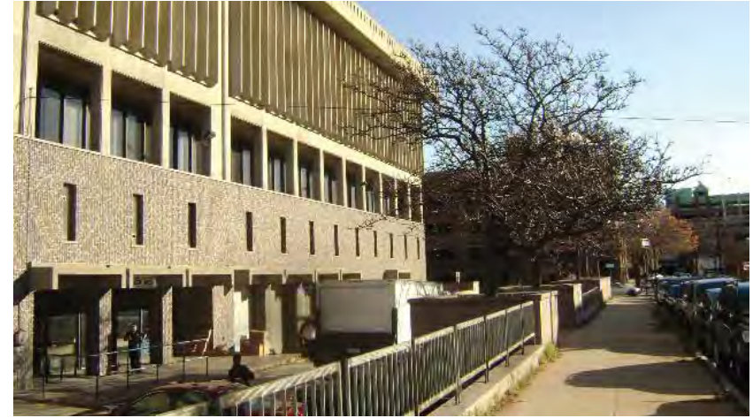
6. VIEW OF SERVICE YARD FROM SPRING ST
