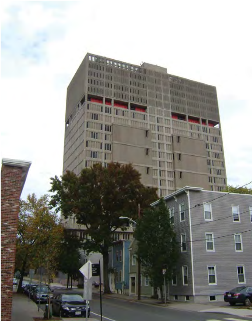
8. VIEW FROM CORNER OF HURLEY ST AND THIRD ST
