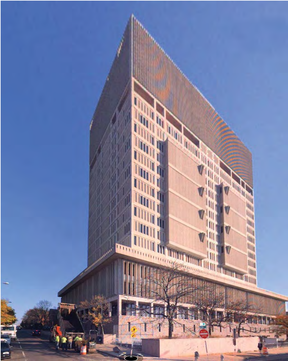
TING PERSPECTIVE – THIRD STREET & SPRING STREET: OVERALL EXISTING BUILDING
