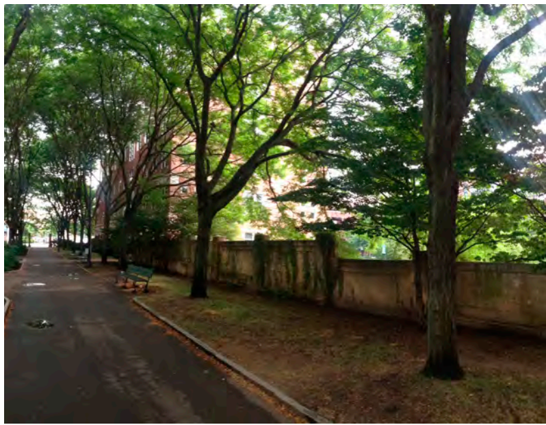
EXISTING RETAINING WALL
