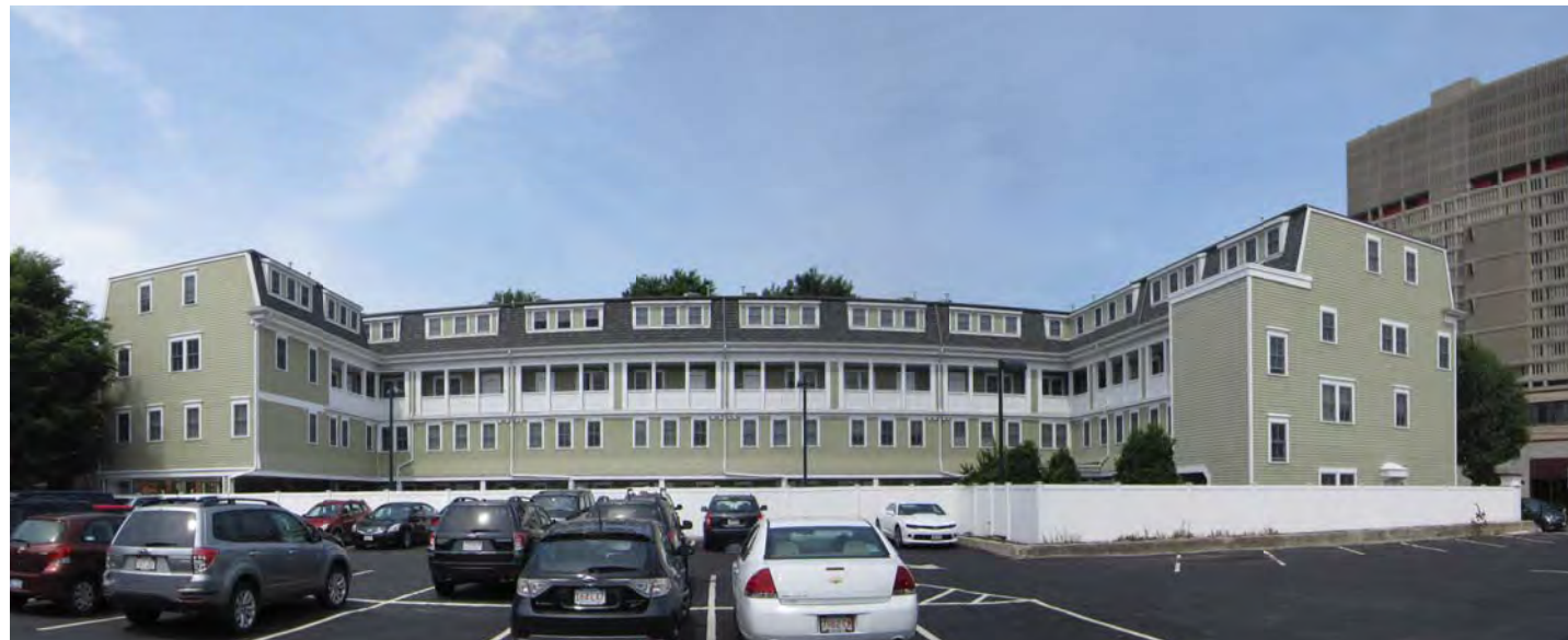
VIEW @ MID BLOCK EXISTING PARKING LOT
