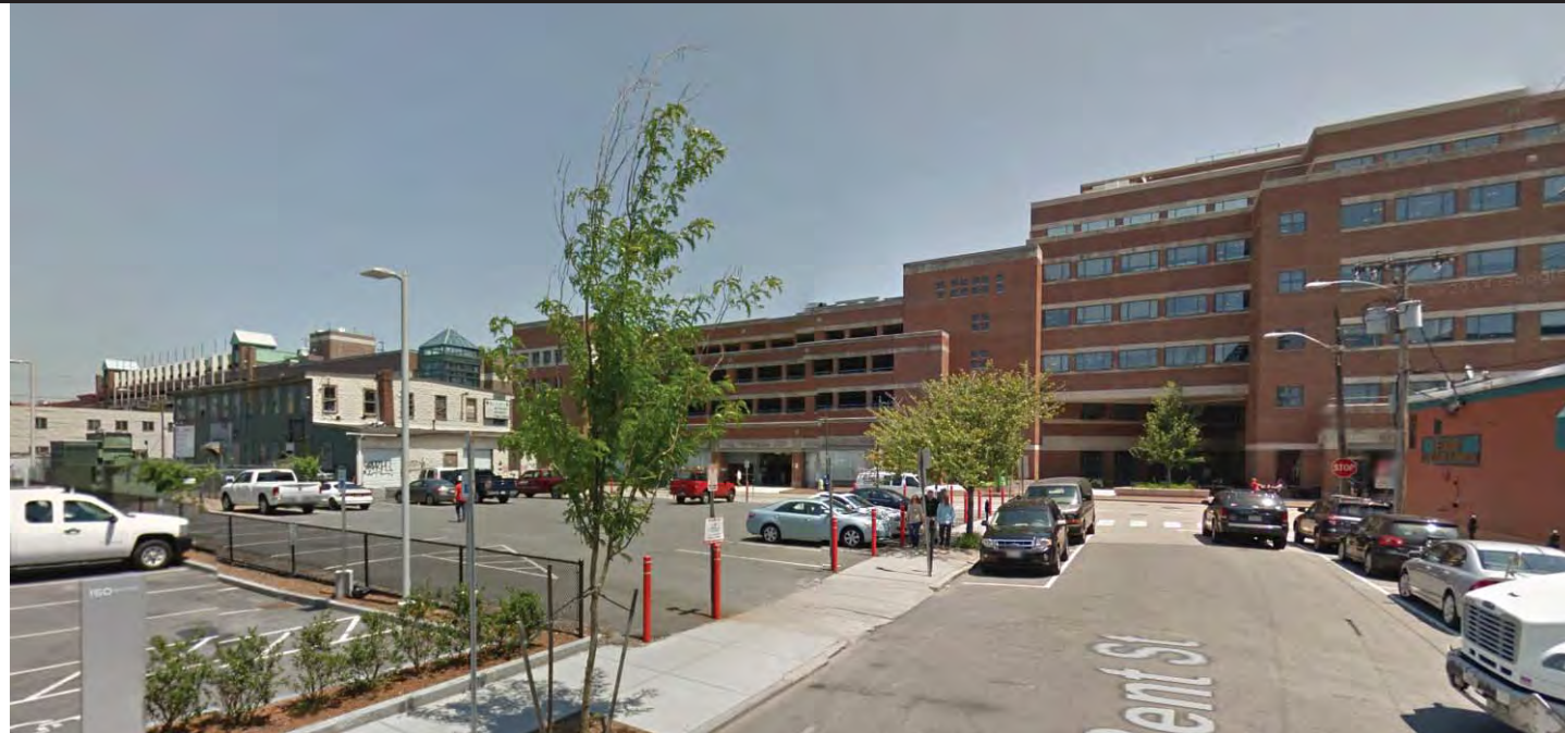
VIEW FROM BENT STREET TO FIRST STREET CORNER
