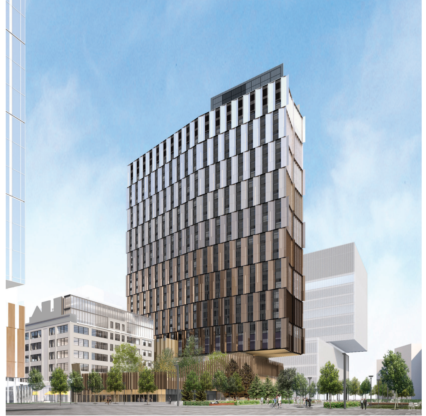
PROPOSED: REVISE PENTHOUSE SCREEN WALL CORRUGATED, ANODIZED ALUMINUM FROM CLEAR ANODIZED TO DEEP BRONZE ANODIZED IN COLOR
