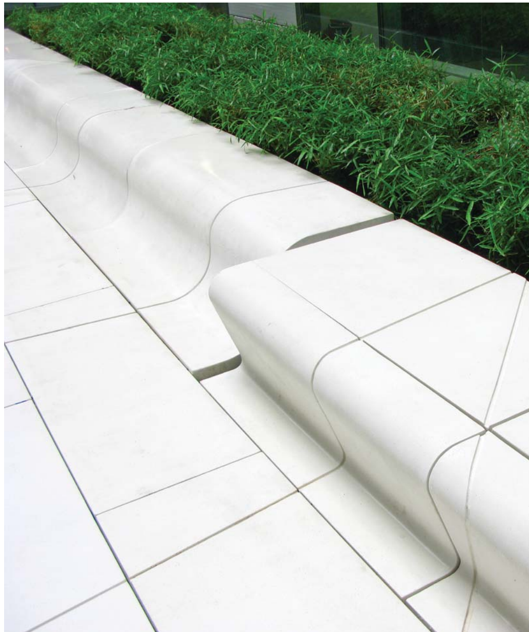
FOLDING PRECAST CONCRETE
