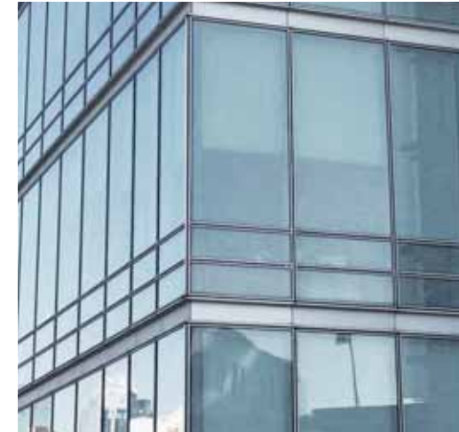
FORMED METAL PANEL AT SLAB (440 HUNTINGTON)
