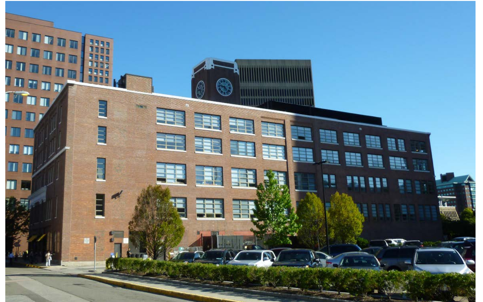
238 MAIN STREET, HAYWARD STREET LOOKING NORTH
