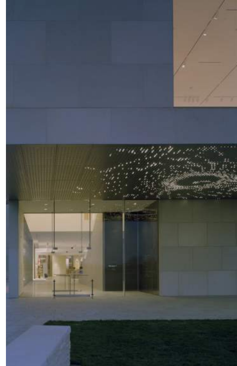
BLDG SOFFIT LIGHTING
