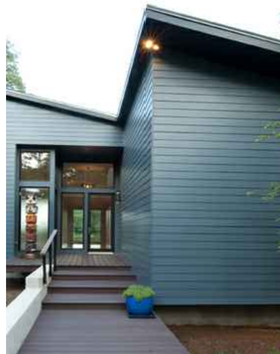
FIBER CEMENT LAP SIDING
