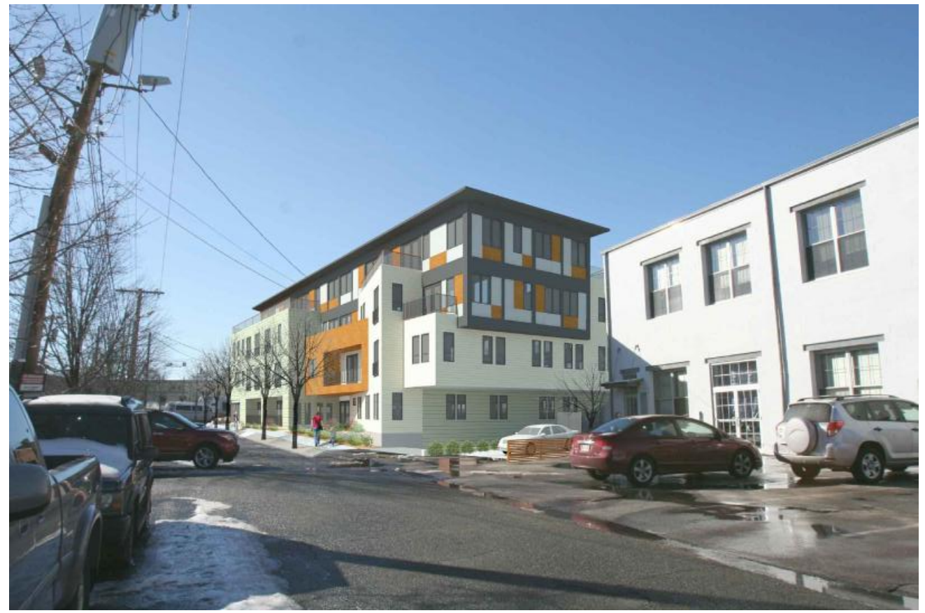
VIEW FROM ELMWOOD STREET
