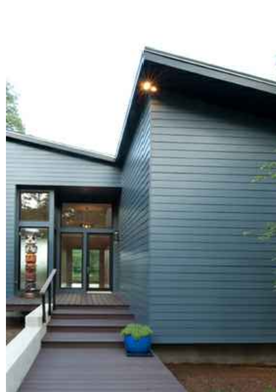
FIBER CEMENT LAP SIDING
