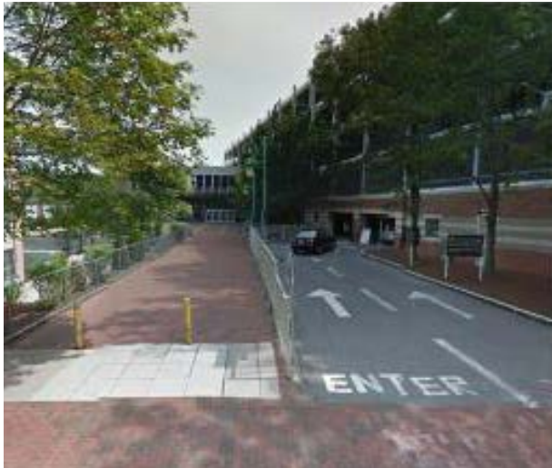
Existing Garage Entrance Driveway & Walk to Cinema Entrance
