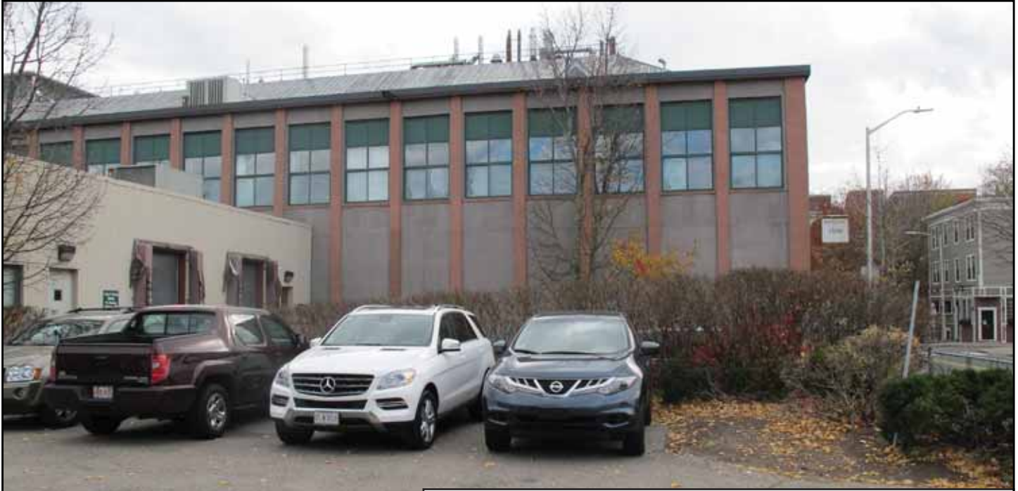
17. View from parking lot towards building #1500
