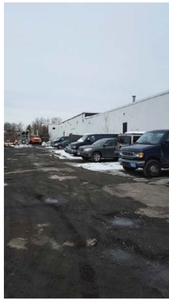
IMAGE 1-5. REAR OF BUILDING AND ABUTTING PROPERTY TO THE WEST
