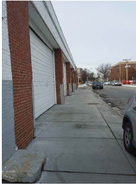
IMAGE 1-1. FRONTAGE ALONG FULKERSON STREET FACING NORTH
