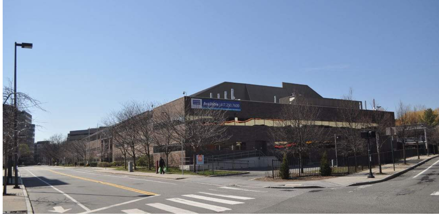
SOUTHEAST CORNER OF SITE
