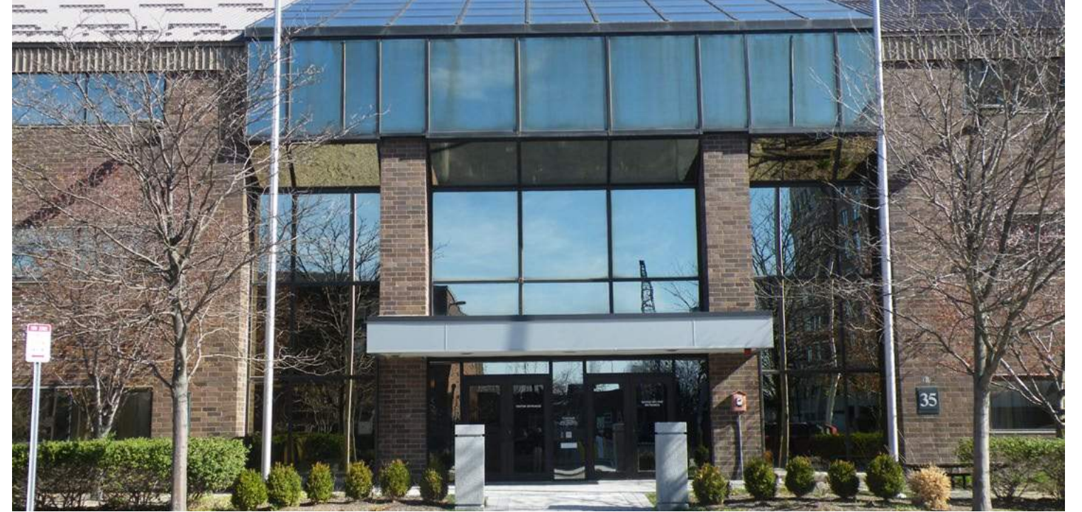
EXISTING MAIN ENTRY
