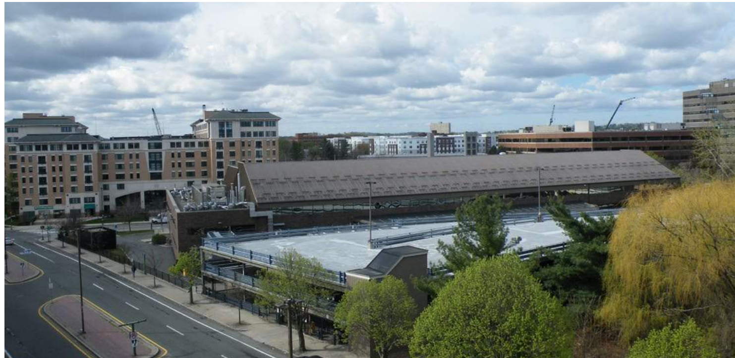
VIEW FROM ALEWIFE GARAGE
