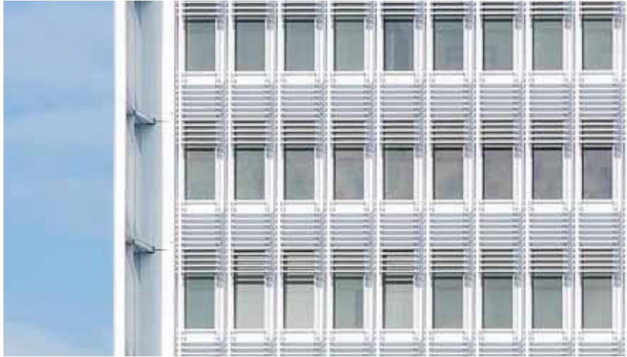
Curtain Wall Panels - Variation in glazing types, frame depths and scales of horizontal and vertical expressions heightens visual interest.
