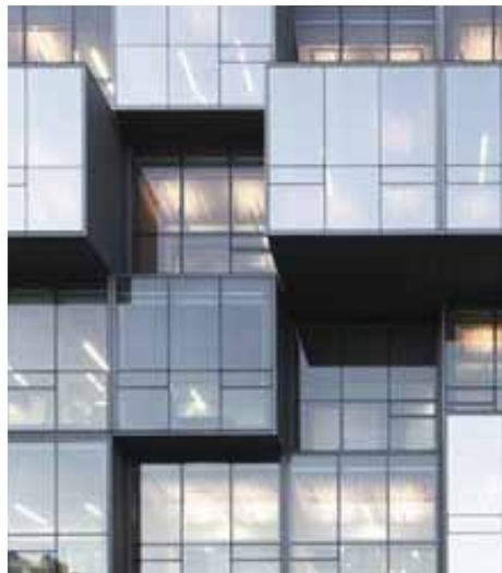
Glazed Volumes - Reveals and recesses in the facade breakdown the proportions of large facades. Plane changes on the facade allow opportunities for exterior spaces and introduce a smaller scale of inhabitation on the facade
