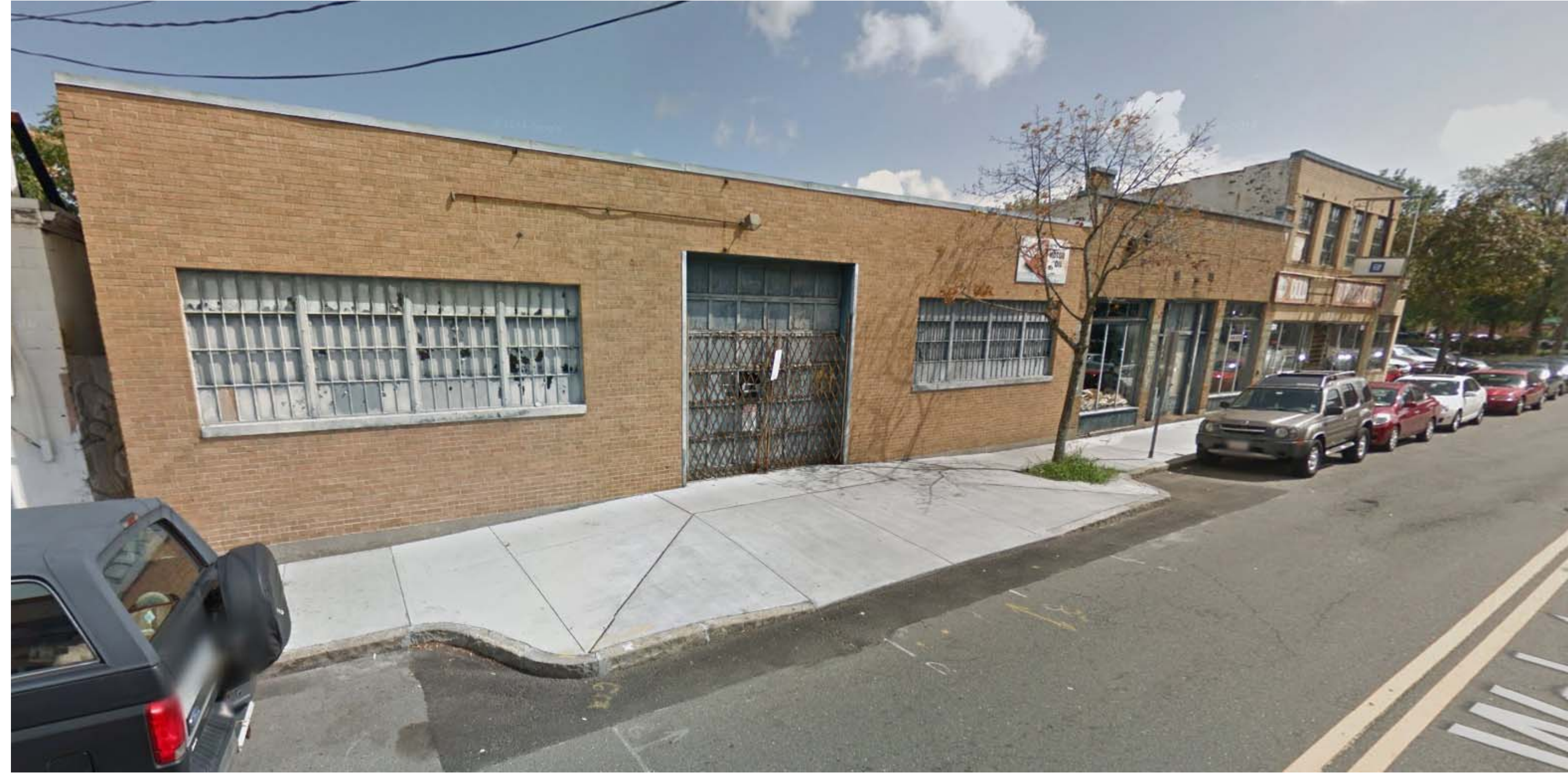
VIEW FROM WEBSTER AVE LOOKING TOWARDS CAMBRIDGE ST
