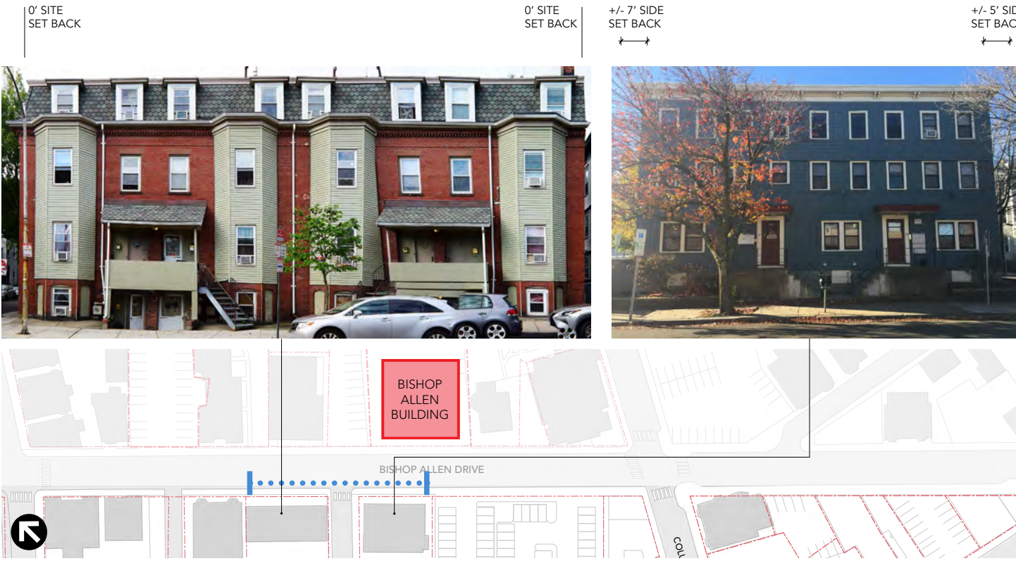
Prepared By: CBT Architects Figure 1.4b Existing Conditions Site Photographs
