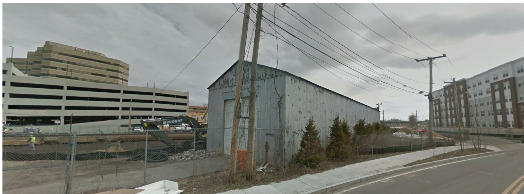
Existing Building from South East
