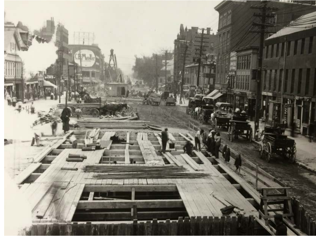
VIEW DOWN MASS AVE - C. 1910
