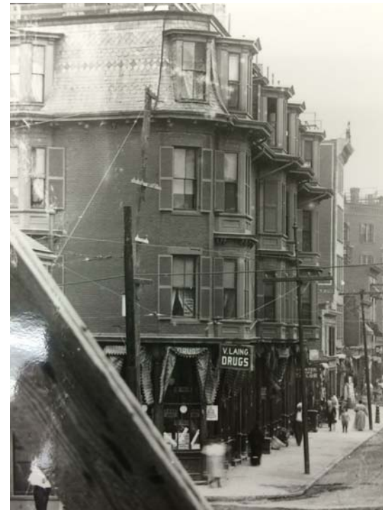
STREET VIEW OF 907 MAIN - C.1915
