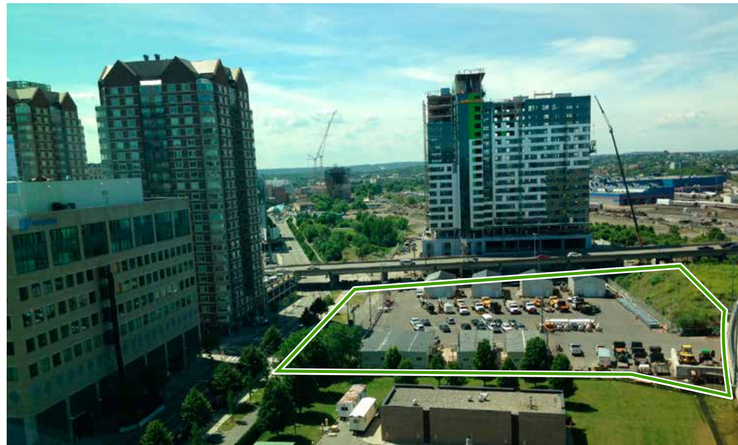
View of the Project Site looking North towards the Twenty/20 Residences
