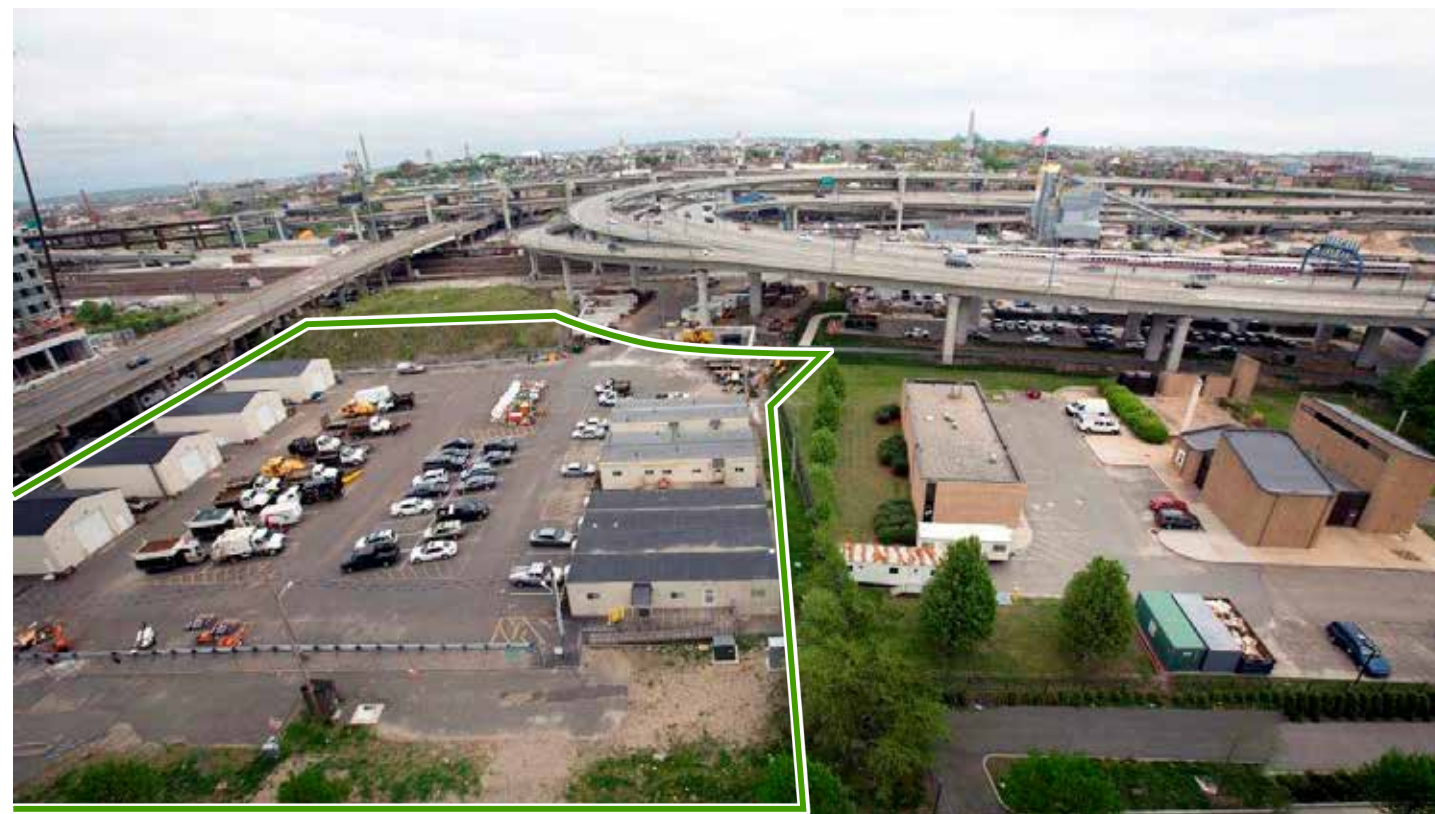
View of the Project to the East looking towards I-93
