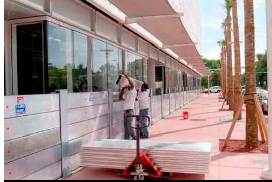
B: Flood Log
