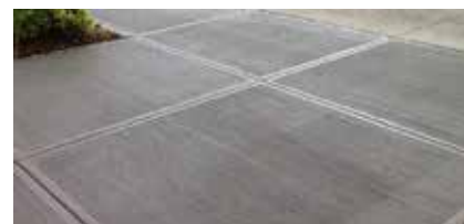
Concrete paving - cast in place
