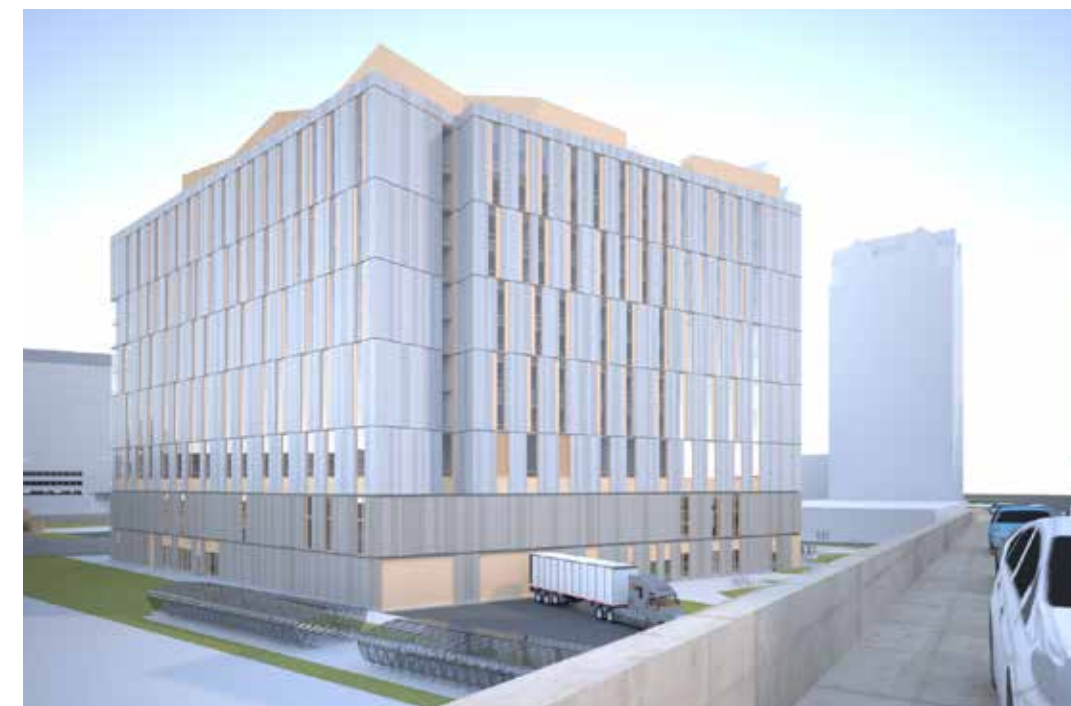
View from the Gilmore Bridge - Original Proposed View
