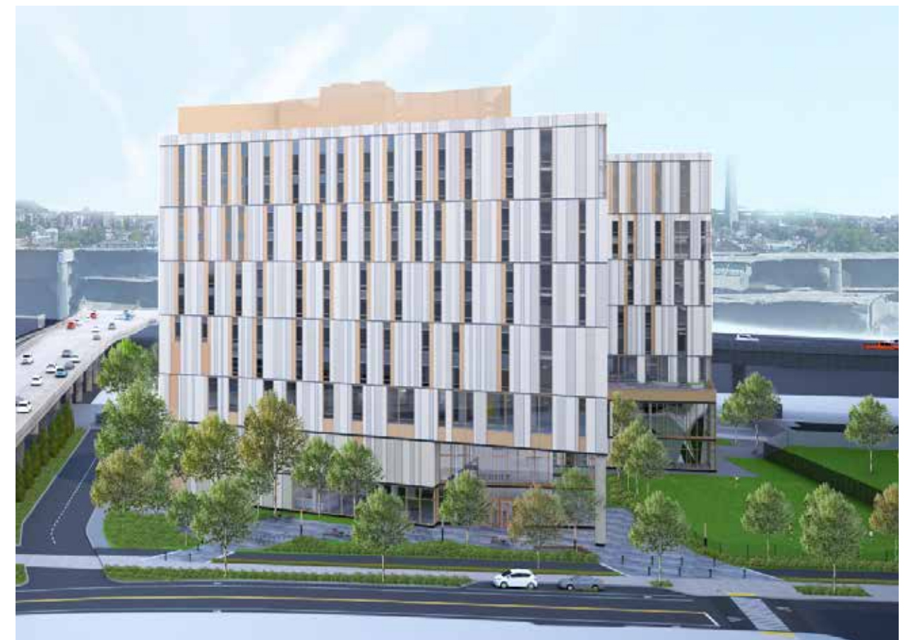
Image 2 - South Elevation View
