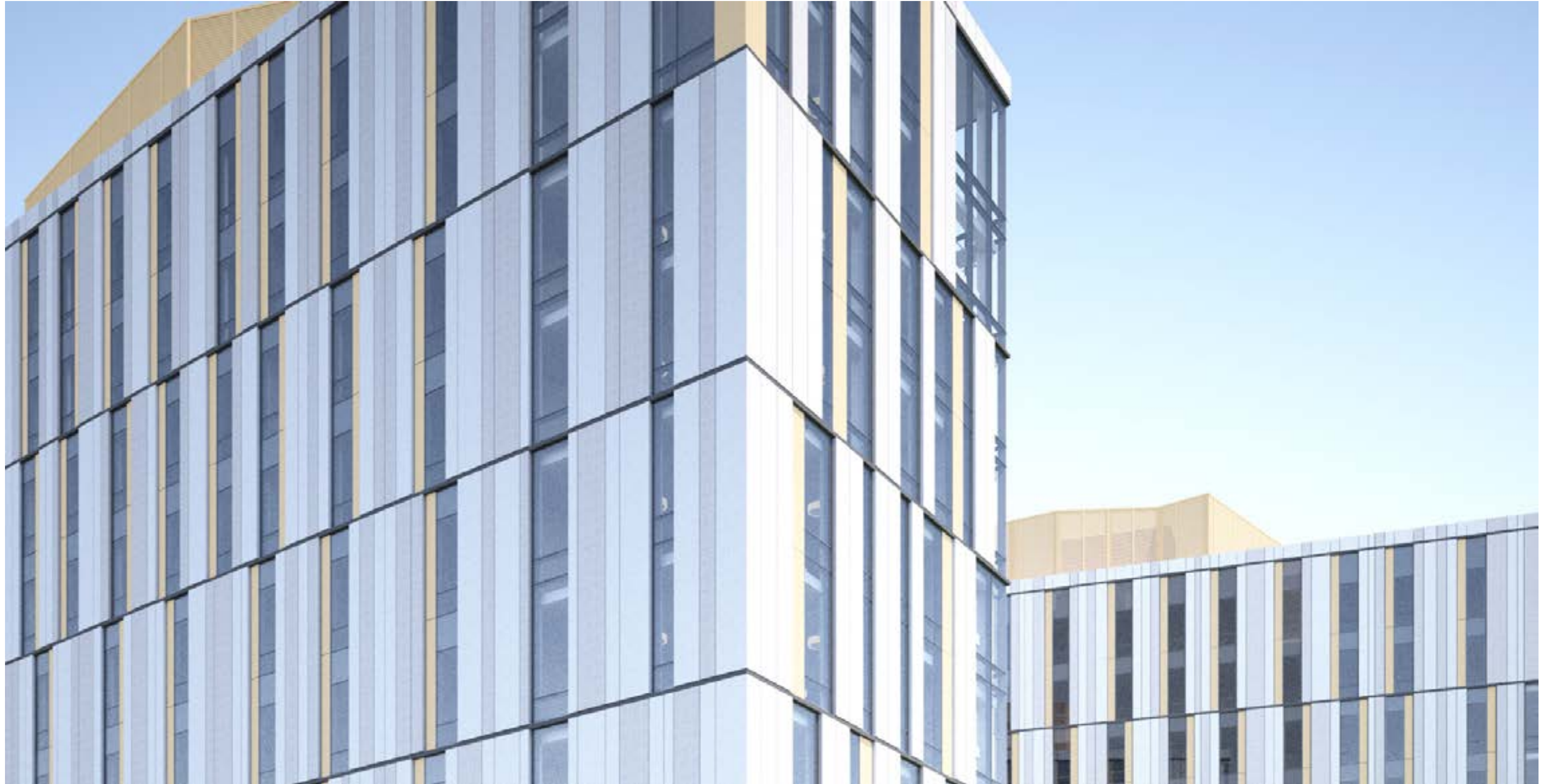
Structurally Glazed Windows with Enhanced Metal Panel Accents
