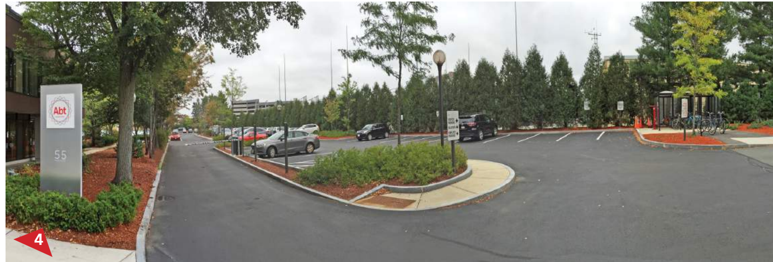
Existing Parking Area Looking North
