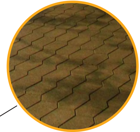
Permeable Paving City Deck \\\ Stoss
