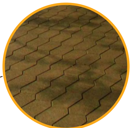
Permeable Paving City Deck \\\ Stoss
