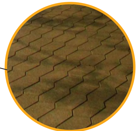
Permeable Paving City Deck \\\ Stoss
