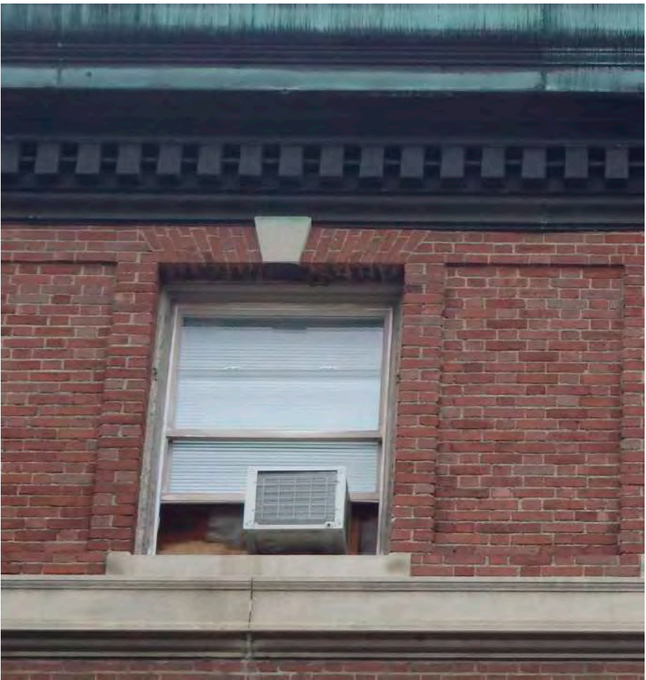
OPEN JOINTS AT LIMESTONE BELT COURSE. COPPER CORNICE TO BE INSPECTED
