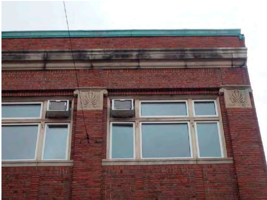
TYPICAL LIMESTONE AND BRICK SOILING
