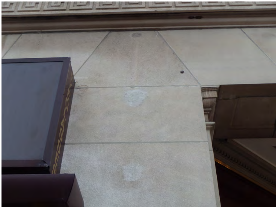
PREVIOUS LIMESTONE PATCHES TO BE REMOVED AND NEW PATCHES INSTALLED TO MATCH SURROUNDING STONE
