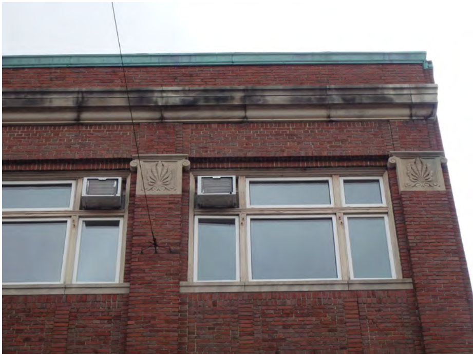
TYPICAL LIMESTONE AND BRICK SOILING
