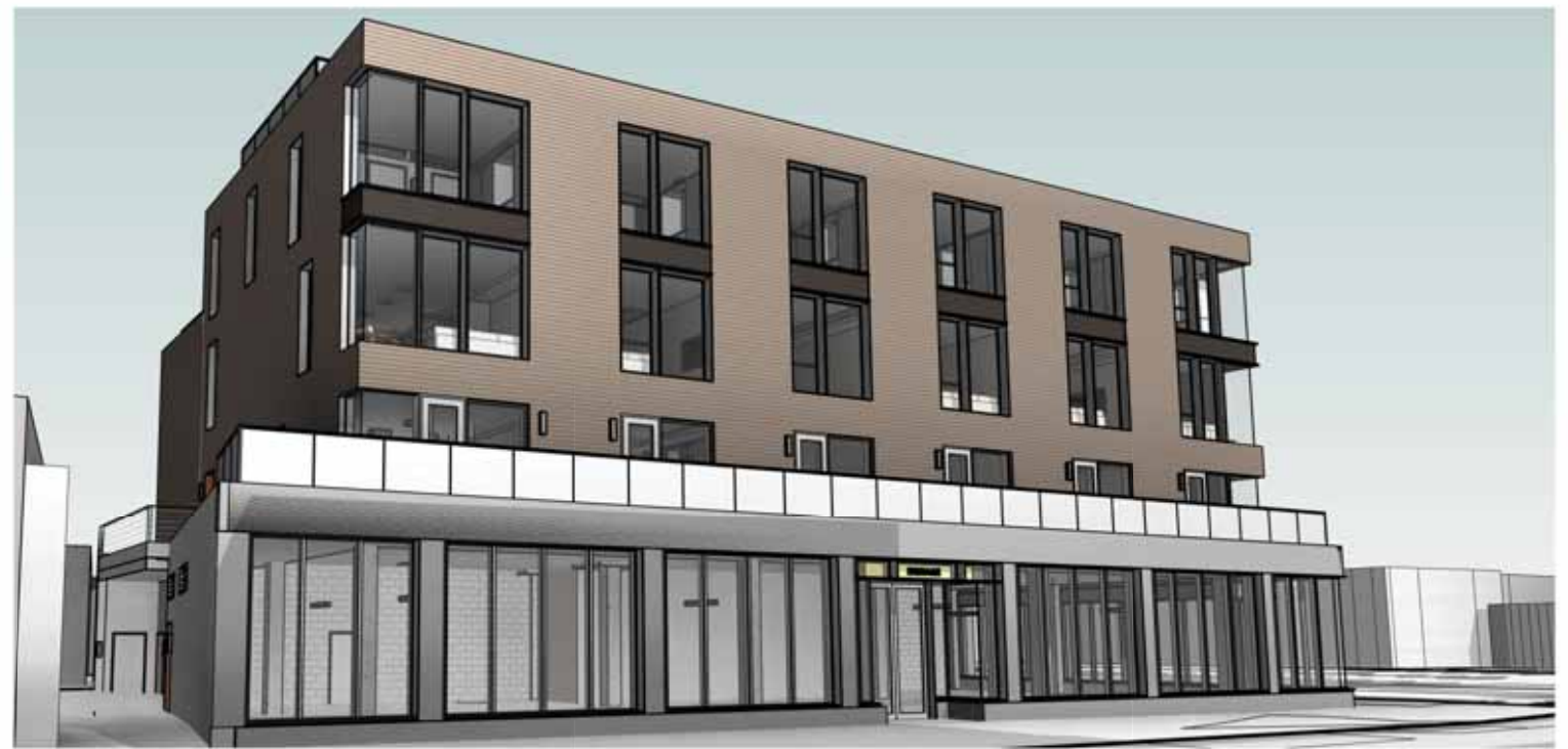
Looking North Across Cambridge St
