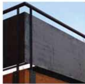
8. Perforated/ Opaque Metal Railing
