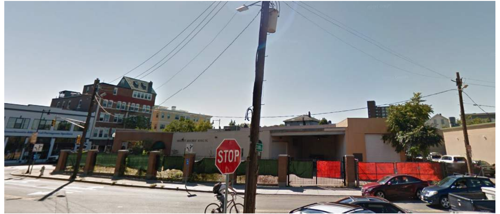
View from Columbia Street
