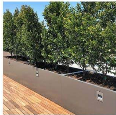
(8) Fiber Cement Clad Planter Box
