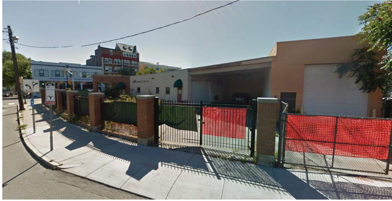
View from Webster Street
