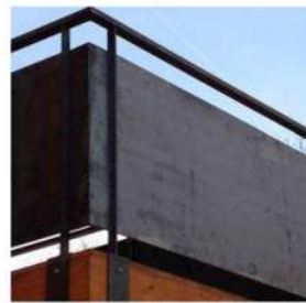
8. Perforated/ Opaque Metal Railing
