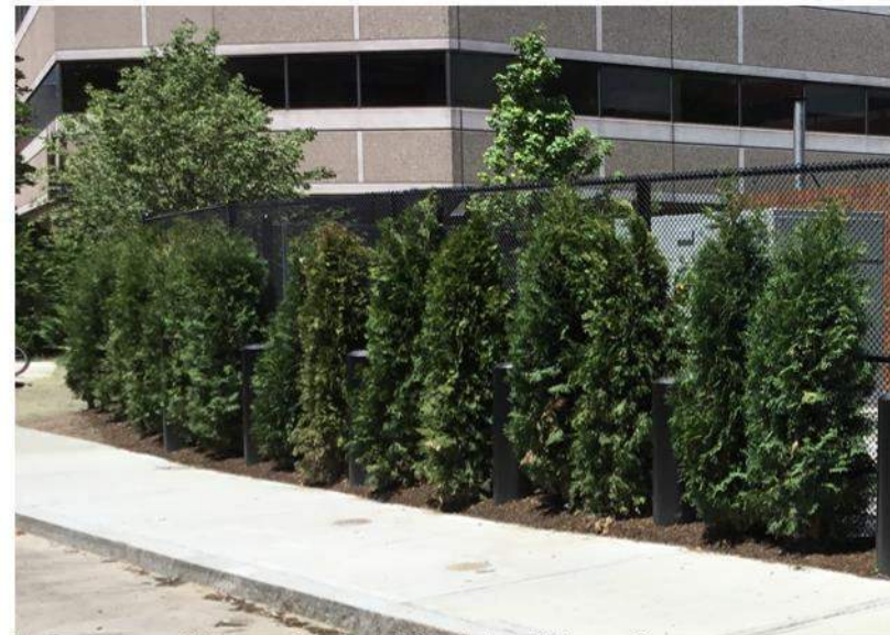
Evergreen Screening at Electrical Transformers
