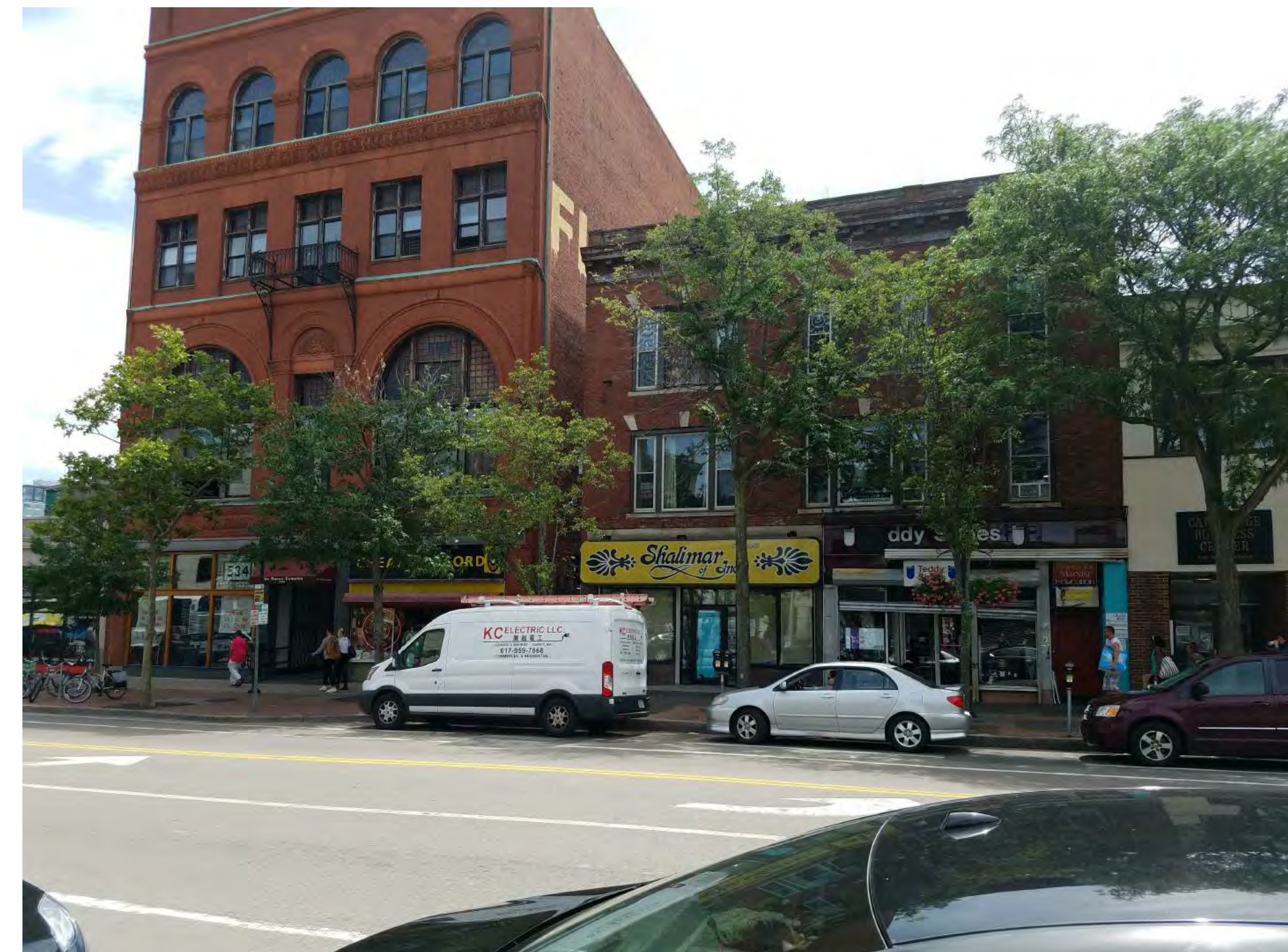
LOOKING SOUTHWEST ACROSS MASS AVE
