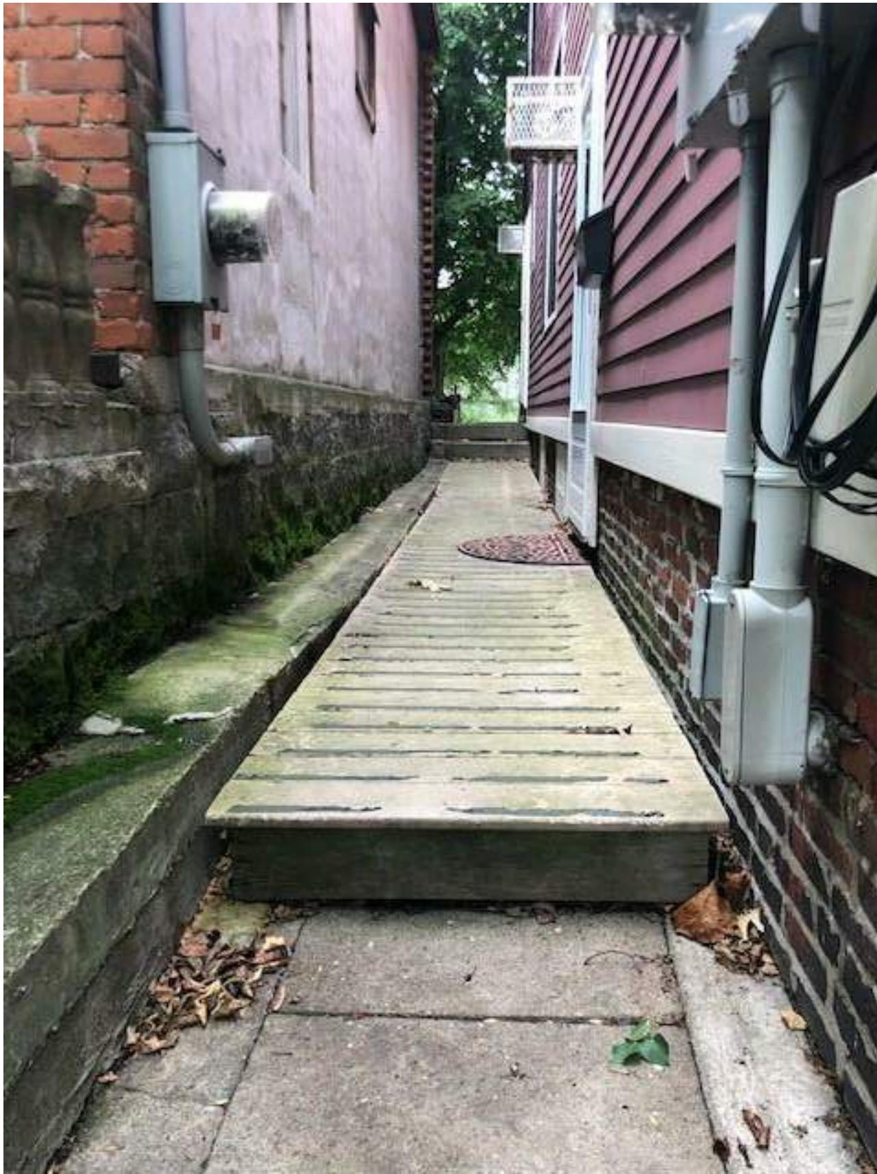
EXISTING WOOD & CONCRETE WALK ALONGSIDE BUILDING (LOOKING TOWARDS REAR)
