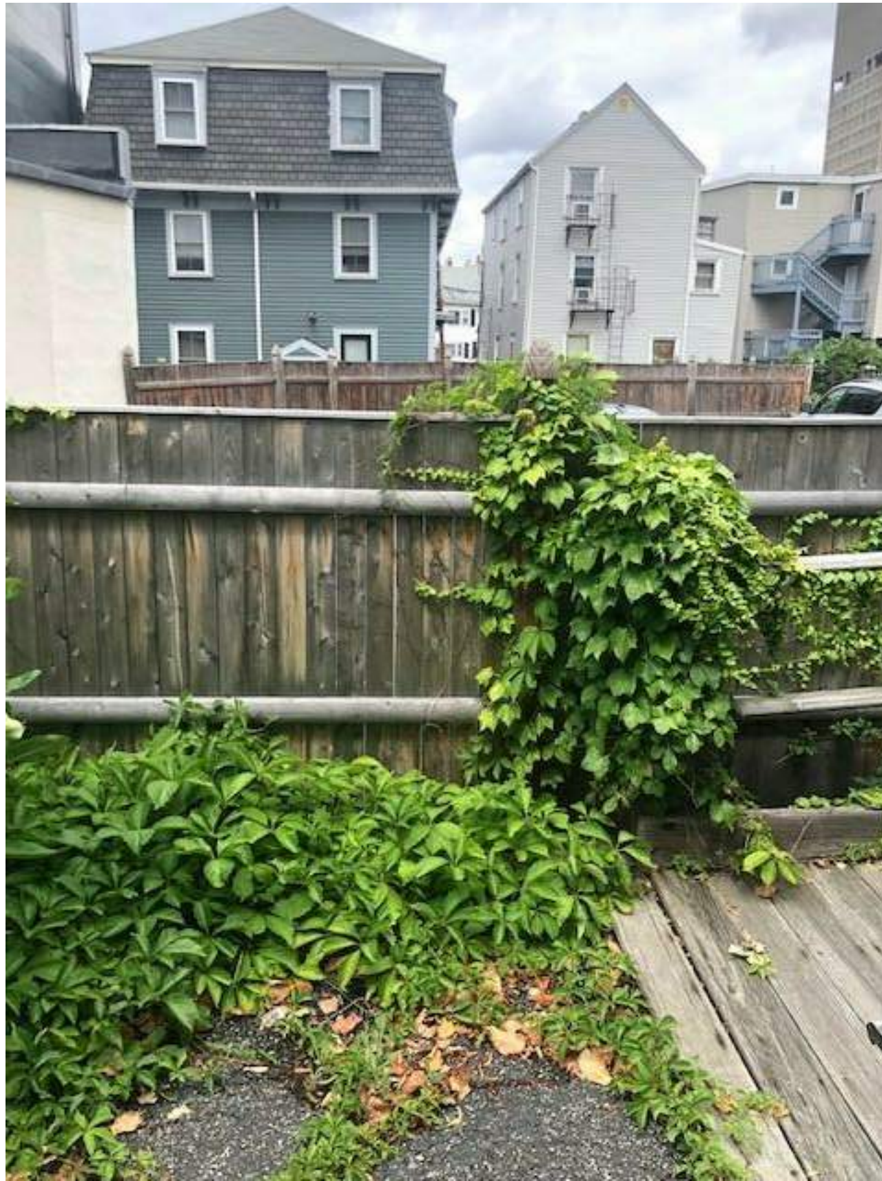
PHOTO OF EXISTING WOODEN FENCE & BASE OF RAMP
