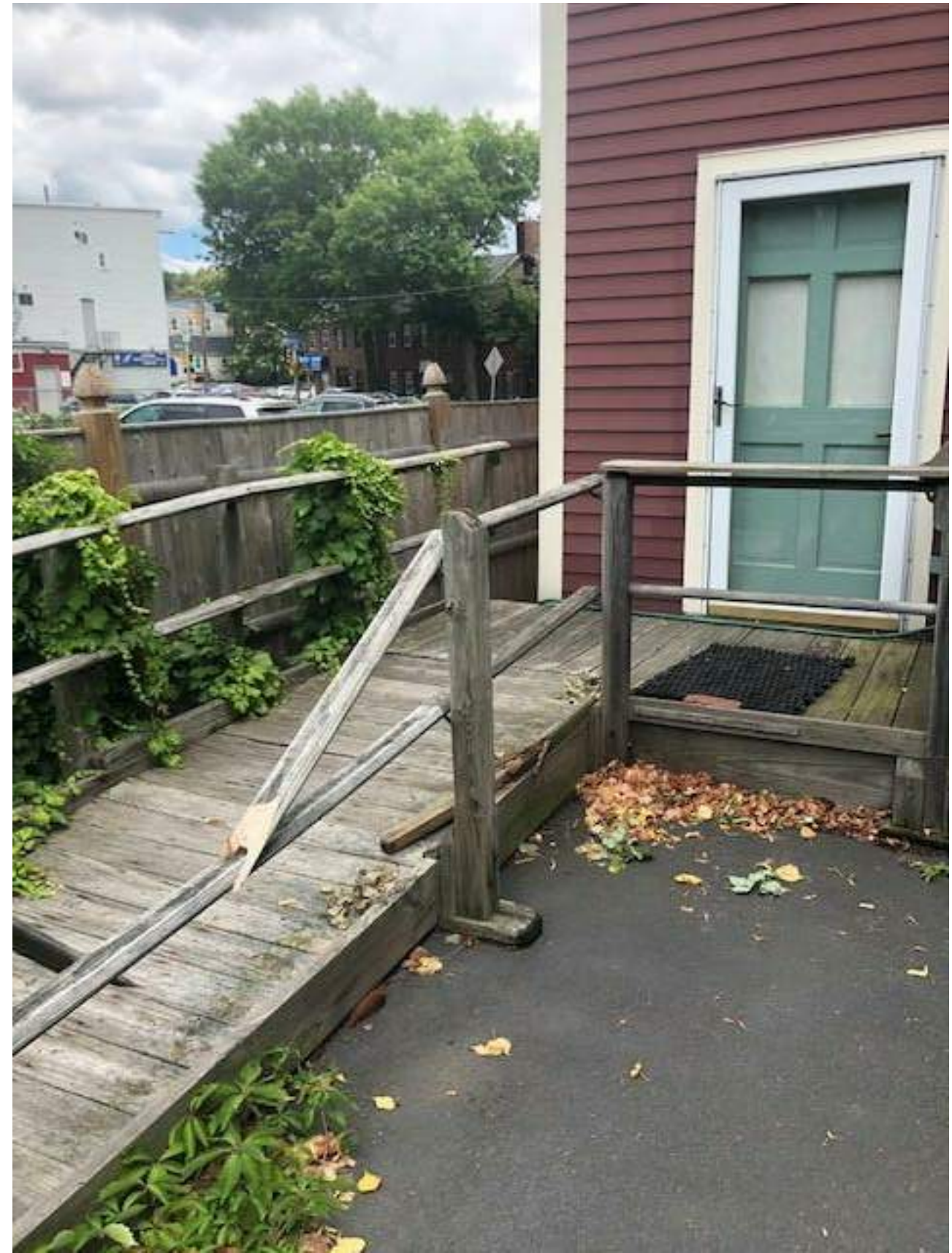
PHOTO OF EXISTING WOOD RAMP, LANDING, & PROPOSED EMPLOYEE ENTRANCE
