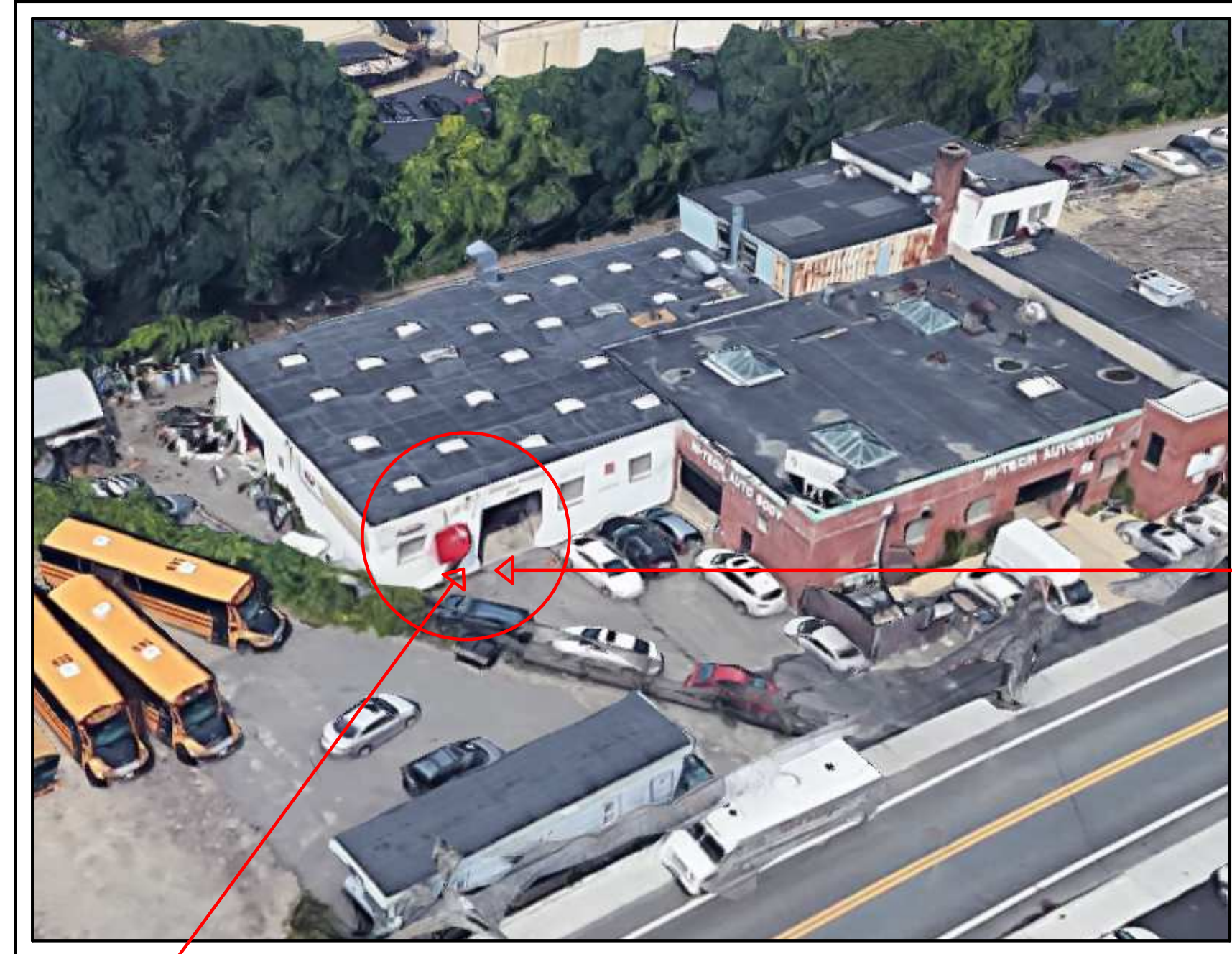
AERIAL FRONT VIEW
