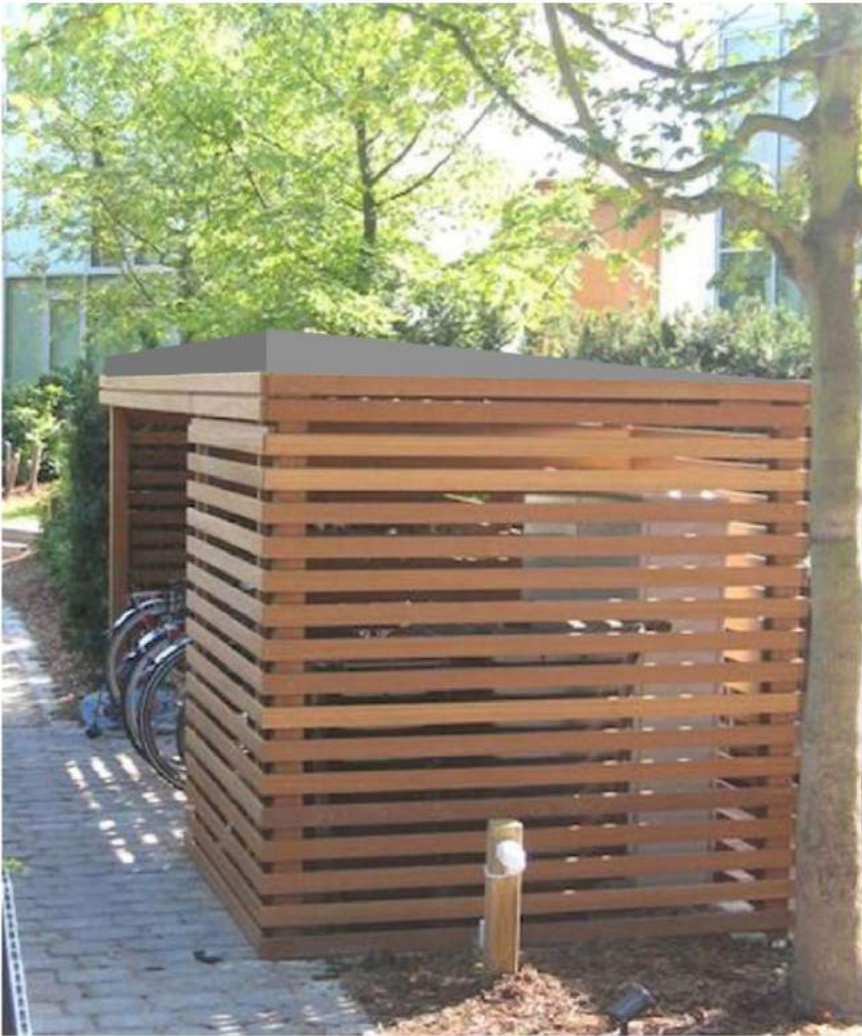
BIKE SHELTER (WOOD SLAT SIDES WITH SIDE AND ROOF WEATHER PROTECTION, SLOPING ROOF, LOCKABLE AND FULLY ENCLOSED FOR 16 BIKES)
