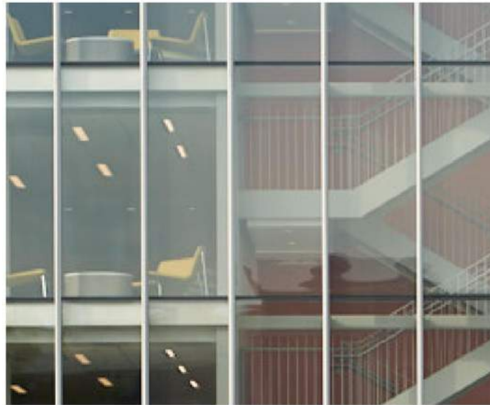
GLAZING: ULTRA LOW IRON GLASS (VITRO STARPHIRE W/ SOLARBAN CTG. OR SIM., VISIBLE LIGHT % TRANSMITTANCE: 74 VISIBLE LIGHT % REFLECTANCE: 11)
